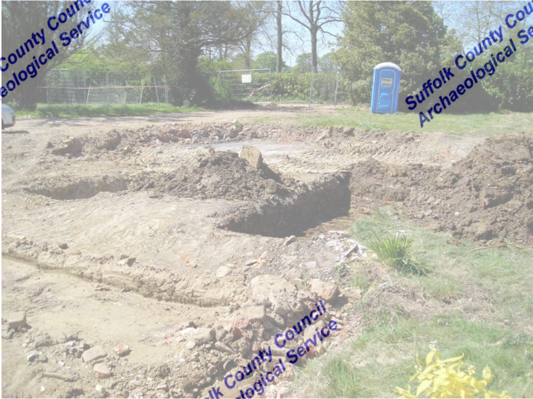
Plate 1: Picture showing north end of Trench 1, Trench 3 and extent of disturbance through former building footprint (looking west)
