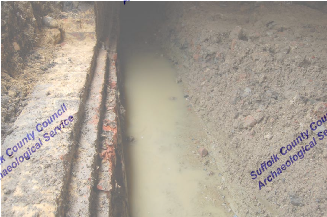
Fig 3: View of the monitored trench on the east side of the barn, looking south
