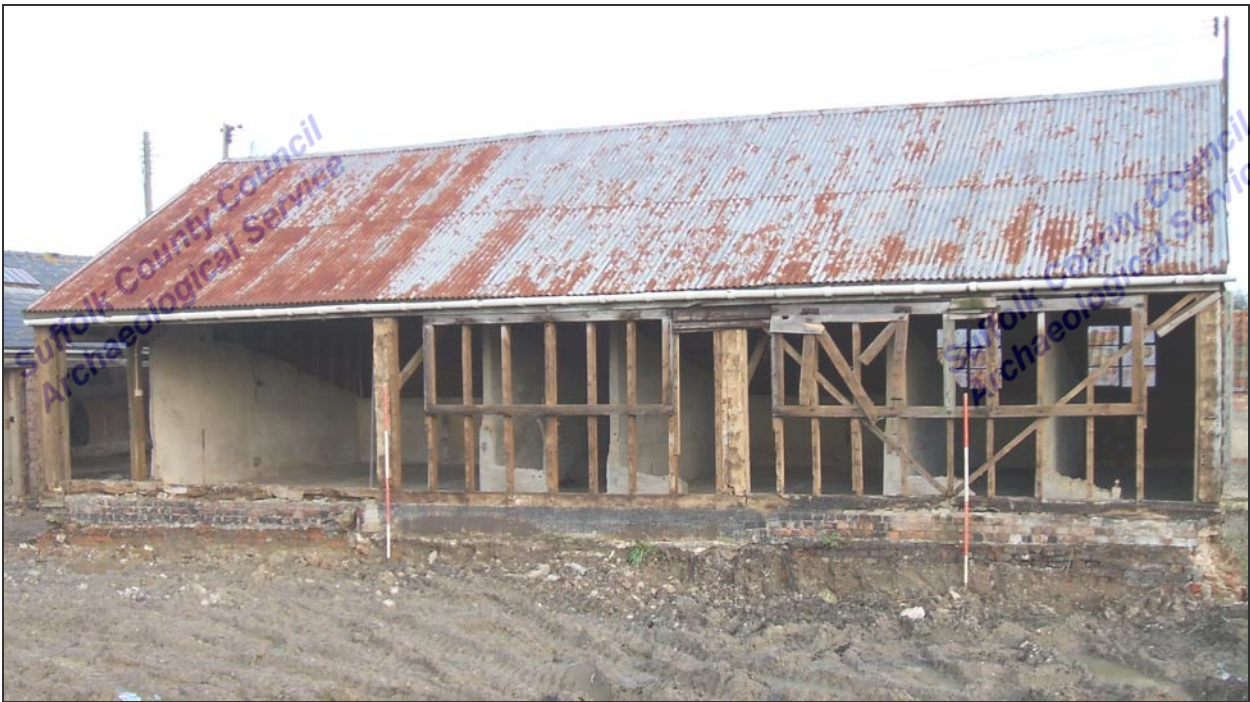
Figure 7. Building 3 West elevation
