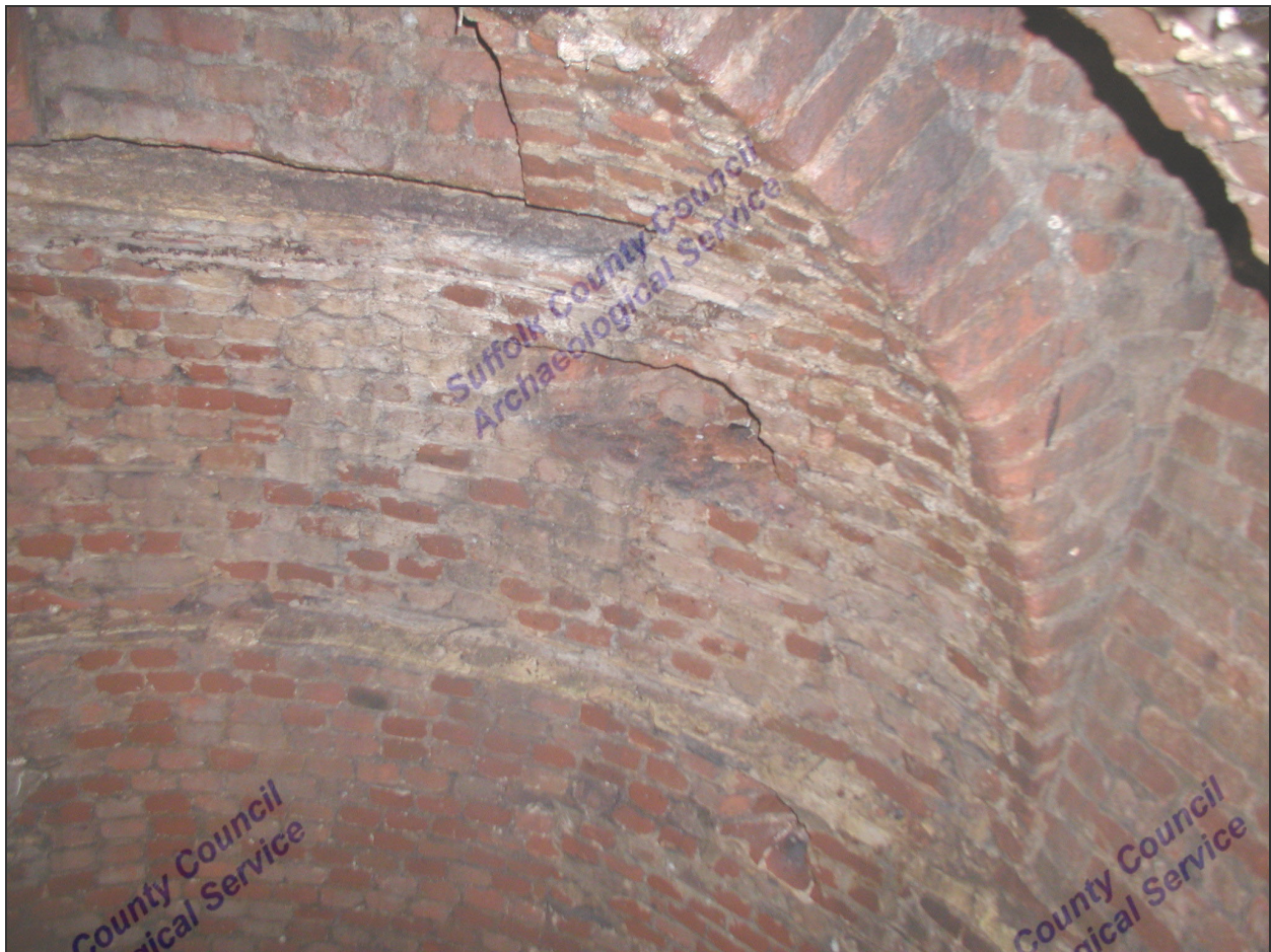
Figure 8. Interior of 0008 icehouse
