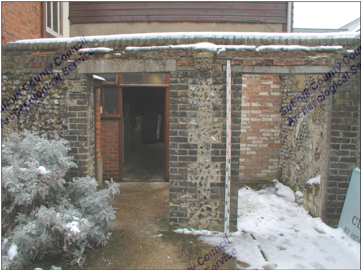
Figure 3. Western face of wall.
