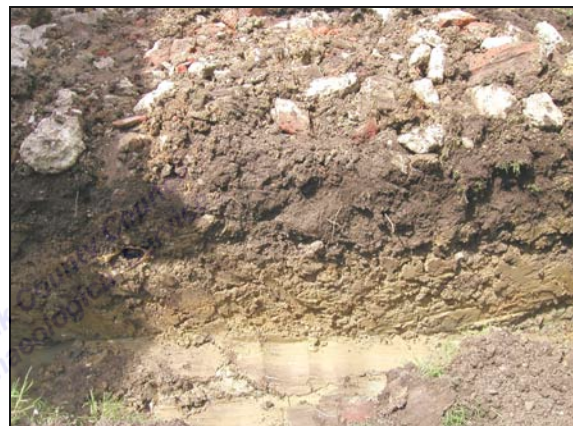
sample of footing trench
