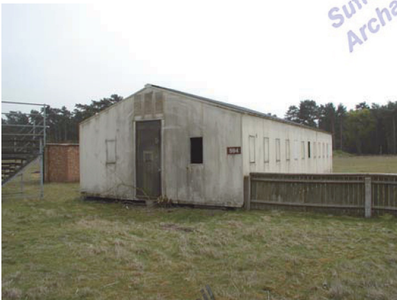
Building 594. View facing SE (P4270057)
