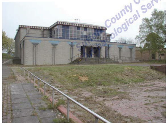
Building 575. View facing E (P4270063)
