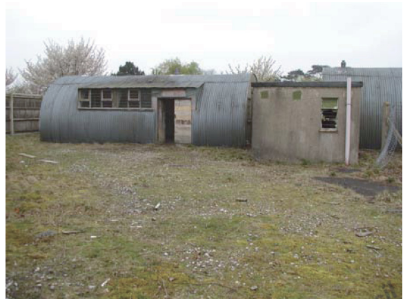
Building 10. View facing NW (P4280038)
