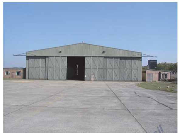
Building 201. View facing E (P4260030)
