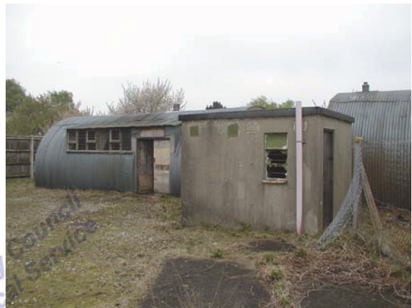
Building 10. View facing NW (P4280039)
