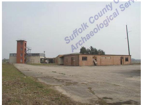
Building 99. View facing N (P4270041)
