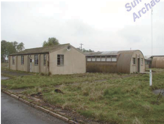
Building 20. View facing SE (P4280013)
