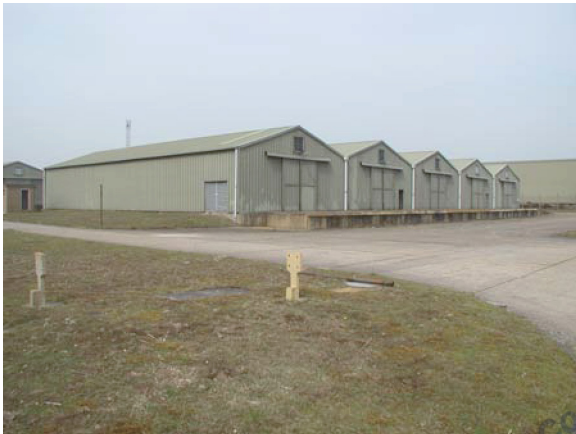
Buildings 224 and 213. View facing NW (P4270050)
