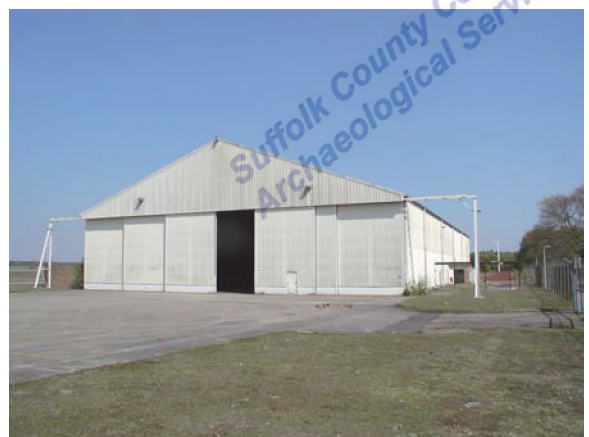
Building 202. View facing E (P4260027)
