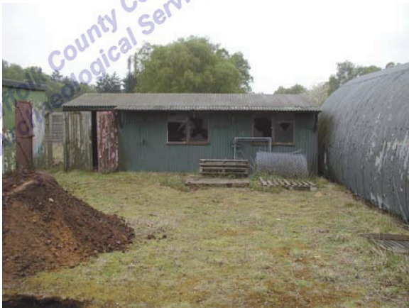
Building 'e'. View facing SW (P4280028)
