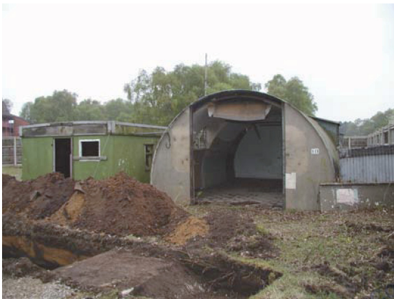
Buildings 'f' and 10. View facing SW (P4280043)
