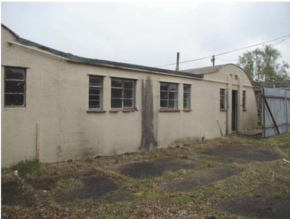
Building 13. View facing SE (P4280021)
