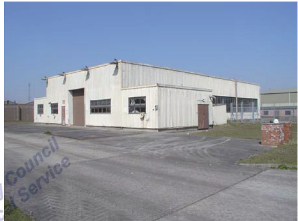
Building 209. View facing NW (P4260007)
