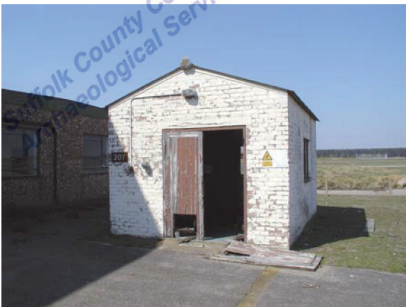
Building 207. View facing N (P4260028)
