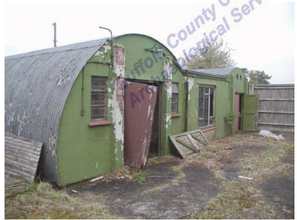
Building 12. View facing NW (P4280026)
