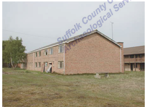
Building 590. View facing NE (P4270075)
