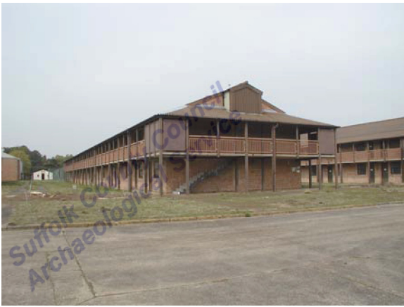
Building 591. View facing NE (P4270073)
