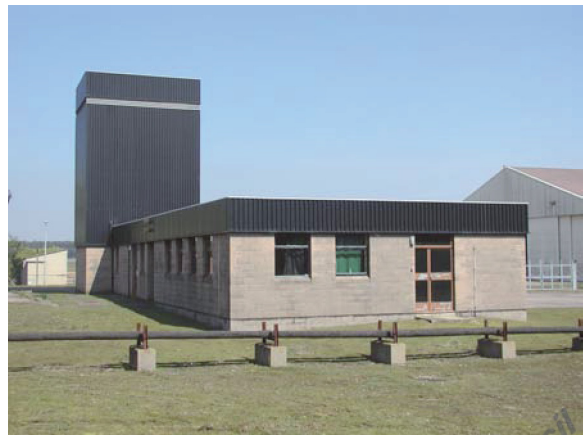
Building 210. View facing N (P4260011)
