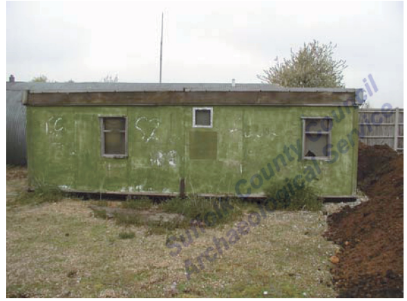
Building 'f'. View facing NW (P4280040)
