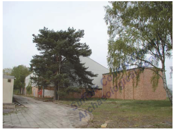
Building 582. View facing NE (P4270077)
