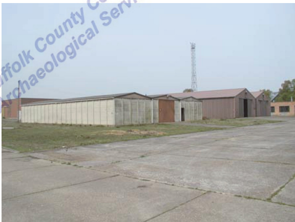
Buildings 218 and 215. View facing NW (P4270052)
