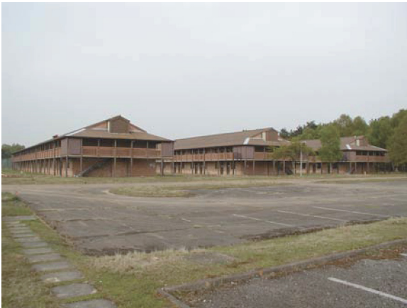
Bldgs 591, 592 and 593. View facing NE (P4270074)
