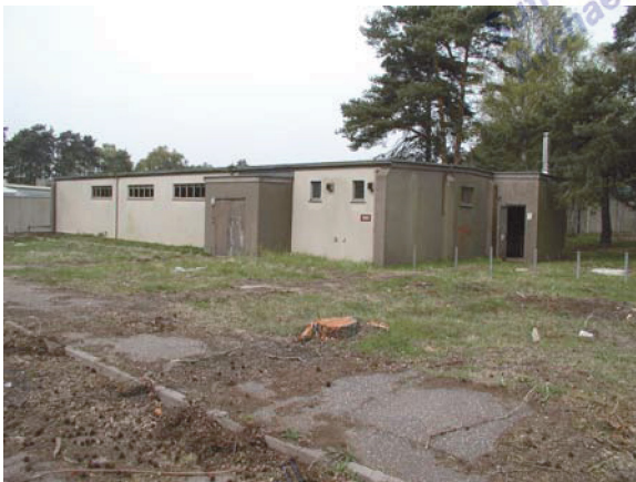
Building 580. View facing N (P4270068)
