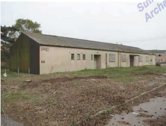
Building 500. View facing E (P4270069)
