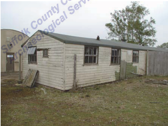
Building 8. View facing S (P4280051)
