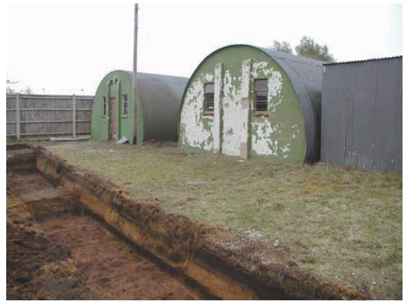
Building 12. View facing N (P4280045)
