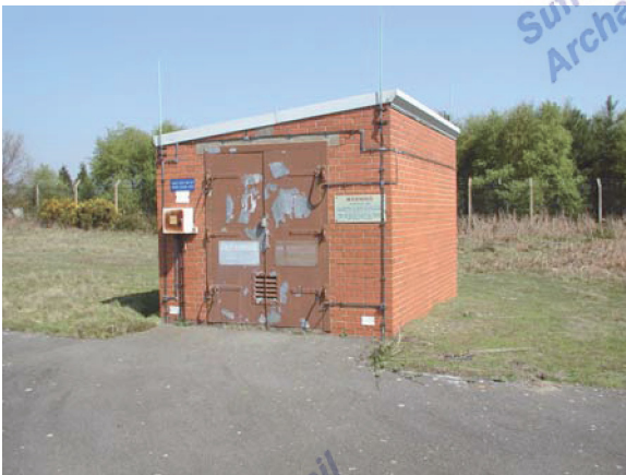
Building 206. View facing NW (P4260026)
