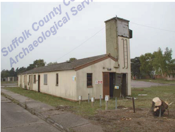
Building 506. View facing N (P4270071)
