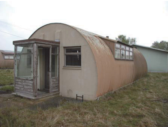
Building 21. View facing NE (P4280005)
