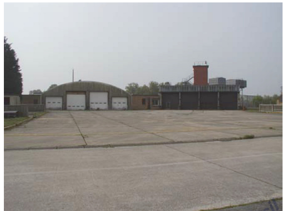
Building 99. View facing S (P4270038)
