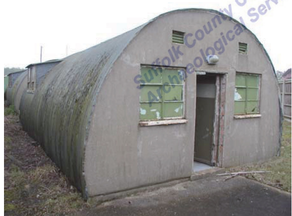
Building 10. View facing NE (P4280036)
