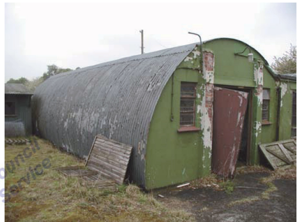
Building 12. View facing NW (P4270027)
