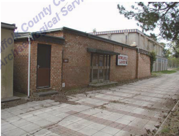
Building 581. View facing NW (P4270066)
