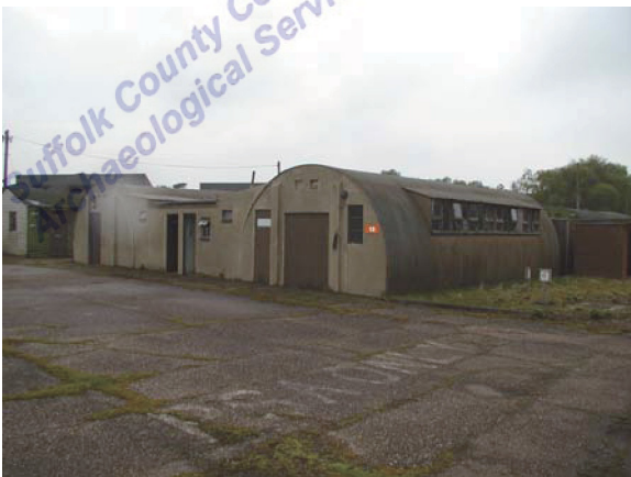
Building 13. View facing S (P4280016)
