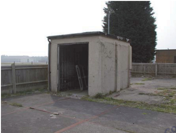
Building 'c'. View facing SE (P4270039)
