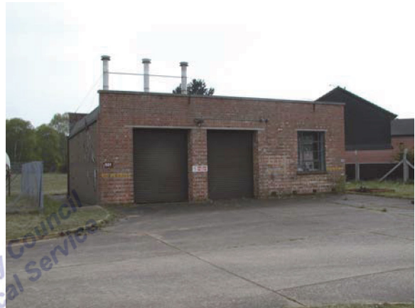
Building 521. View facing SW (P4270072)
