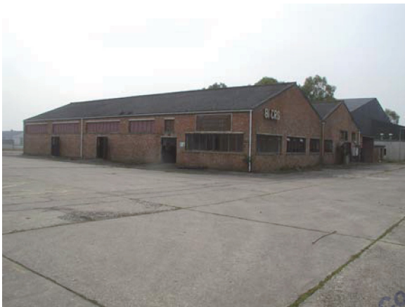
Building 111. View facing SE (P4270042)
