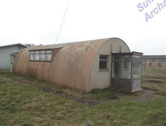
Building 21. View facing SE (P4280006)
