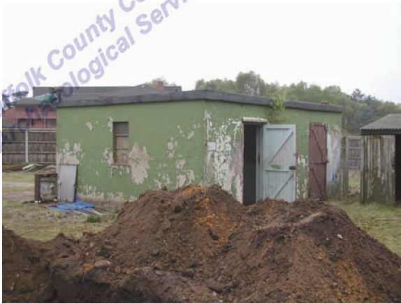
Building 11. View facing SW (P4280029)
