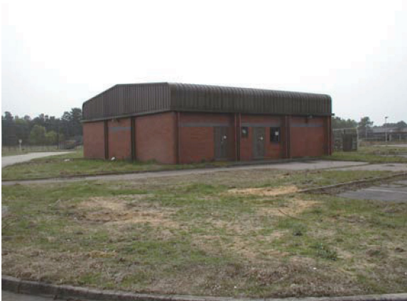
Building 6. View facing S (P4270056)
