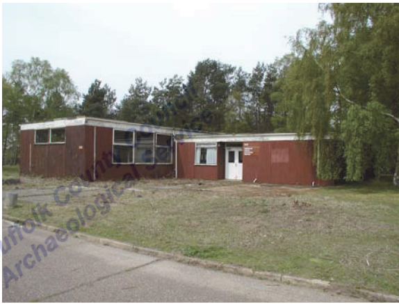
Building 576. View facing NW (P4270062)
