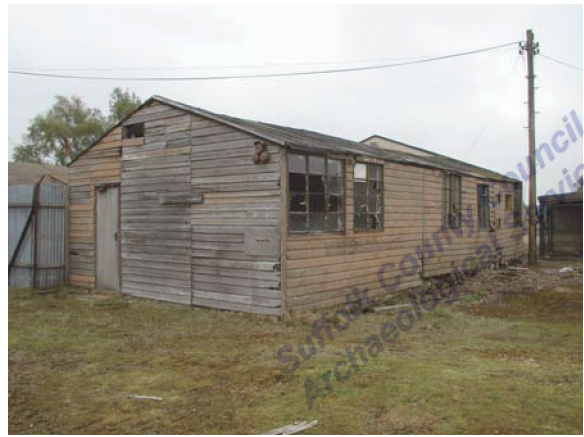
Building 14. View facing NE (P4280048)
