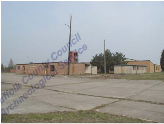
Building 99. View facing NW (P4270040)
