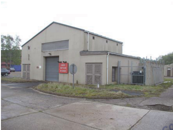
Building 16. View facing SW (P4280014)
