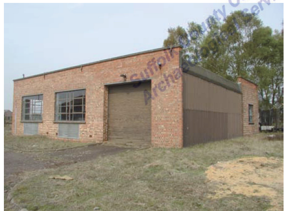
Building 211. View facing NW (P4270053)
