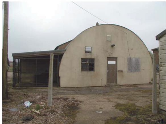
Building 15. View facing NE (P4280054)
