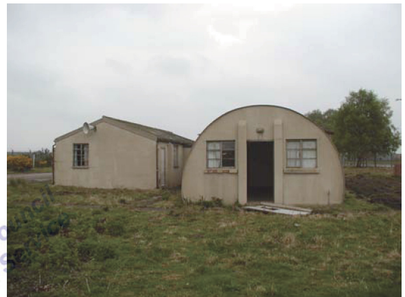
Building 20. View facing NE (P4280010)
