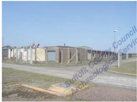
Building 208. View facing NW (P4260012)
