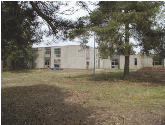
Building 579/580. View facing E (P4270078)
