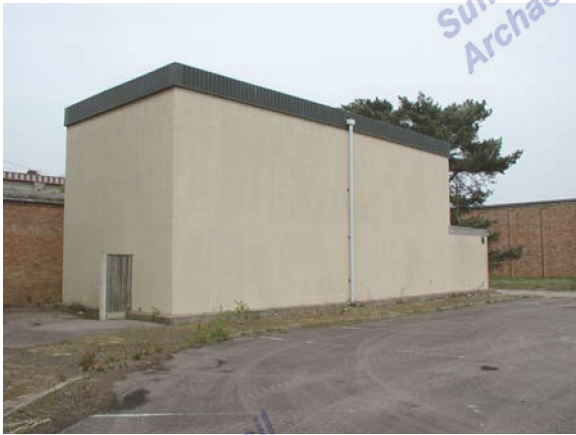
Building 'd'. View facing NE (P4270067)
