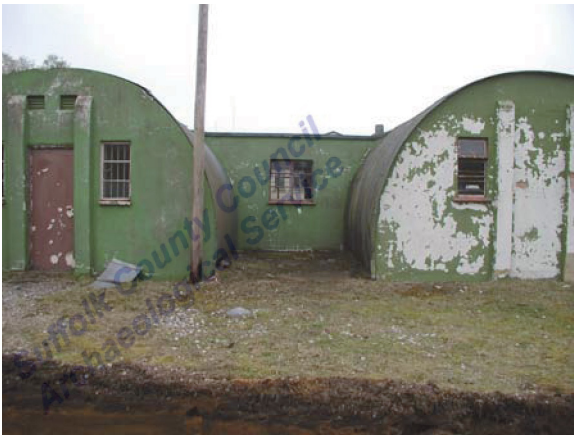
Building 12. View facing NE (P4280046)
