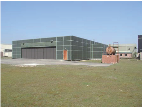
Building 205. View facing NW (P4260008)
