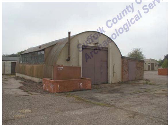
Building 15. View facing NW (P4280056)
