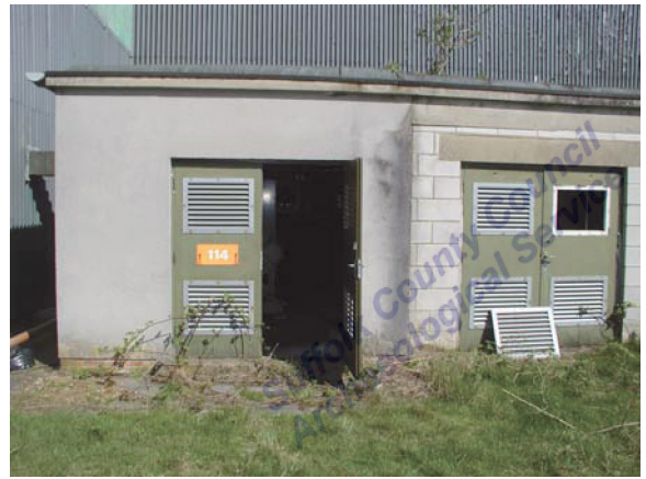
Building 114. View facing E (P4260037)
