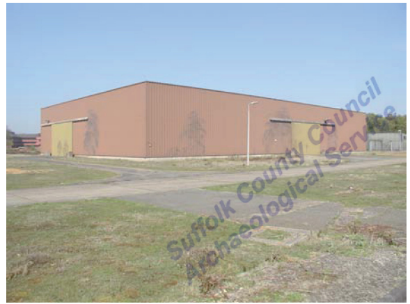
Building 219. View facing NW (P4260001)
