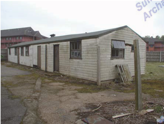
Building 8. View facing S (P4280050)
