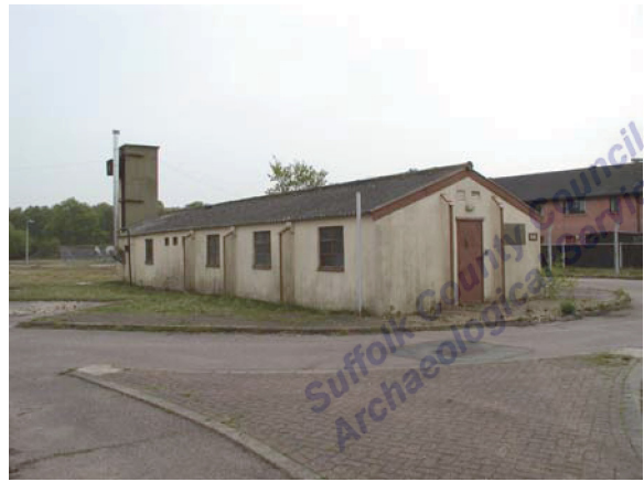
Building 506. View facing S (P4270070)
