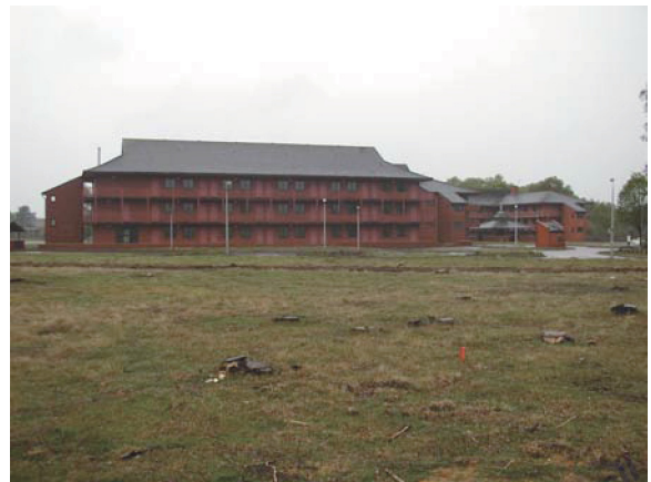
Building 600. View facing SW (P4280003)
