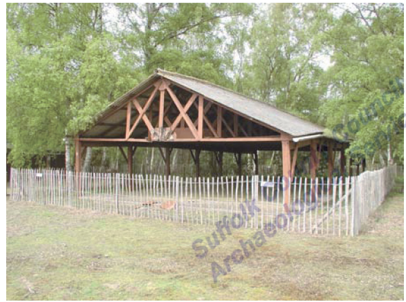
Building 597. View facing NW (P4270061)
