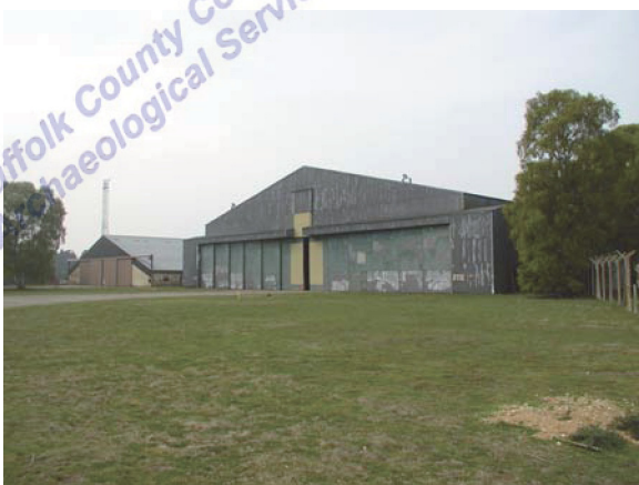
Buildings 113 and 115. View facing SW (P4270044)
