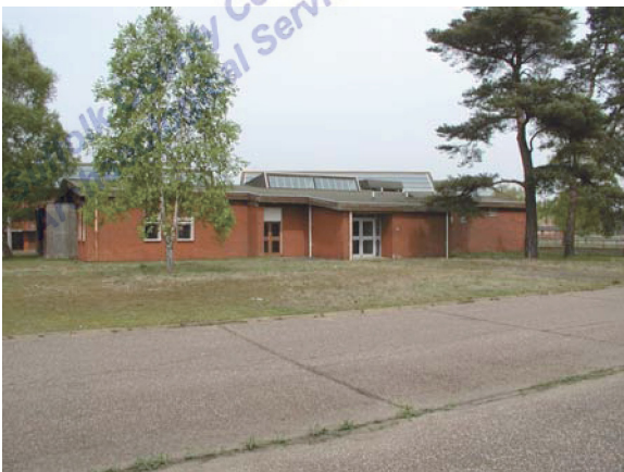
Building 596. View facing NE P4270060)
