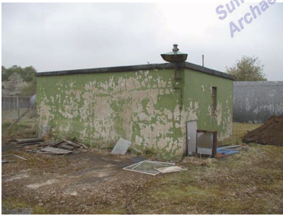
Building 11. View facing NW (P4280033)
