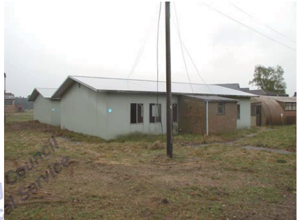
Buildings 30 and 29. View facing SW (P4280002)
