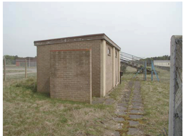
Building 585. View facing NE (P4270059)
