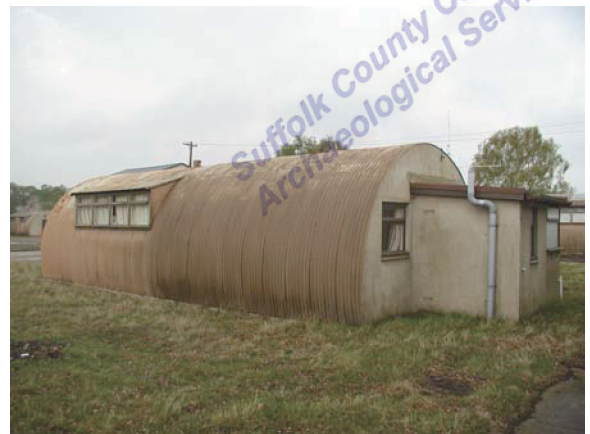
Building 21. View facing NW (P4280008)
