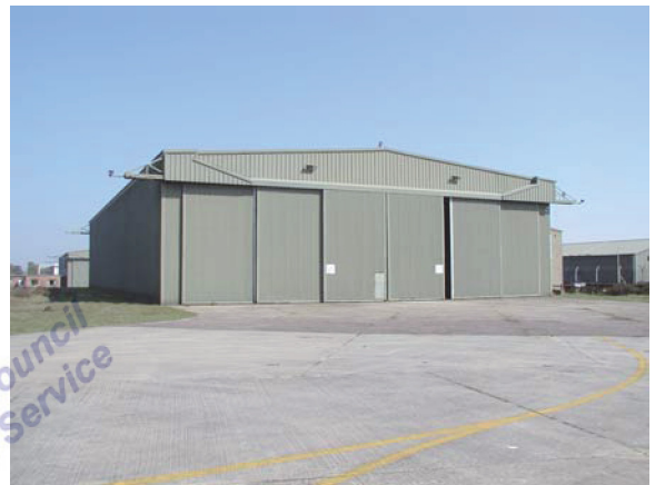
Building 200. View facing SE (P4260034)
