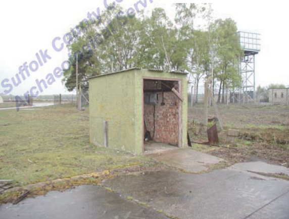
Building 28 (?). View facing NE (P4280001)
