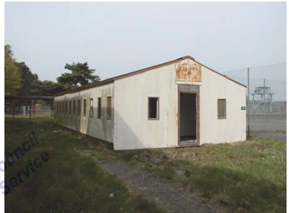
Building 583. View facing NE (P4270076)
