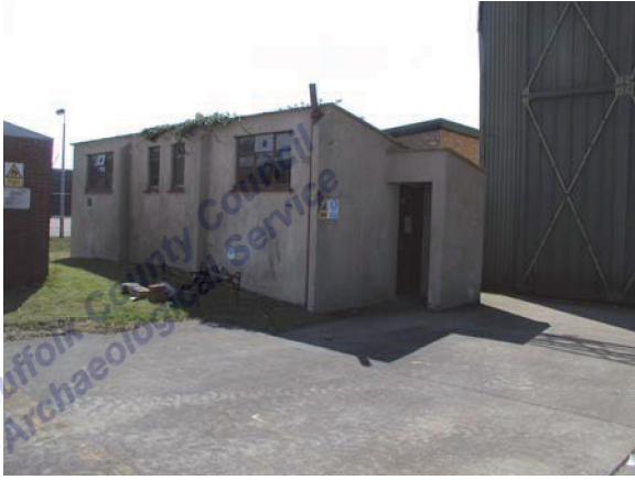
Building 'b'. View facing SW (P4260029)
