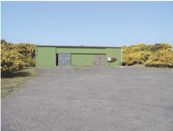
Building 247. View facing W (P4260005)
