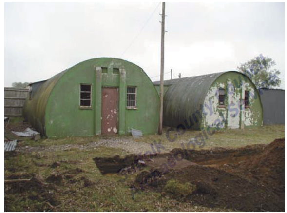
Building 12. View facing E (P4280044)
