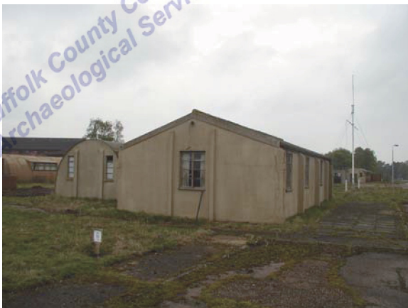
Building 20. View facing SW (P4280012)
