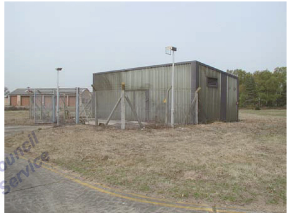
Building 220. View facing NW (P4270054)
