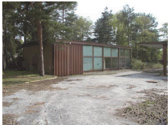
Building 566. View facing SW (P4270079)
