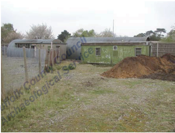
Buildings 10 and 'f'. View facing NW (P4280047)
