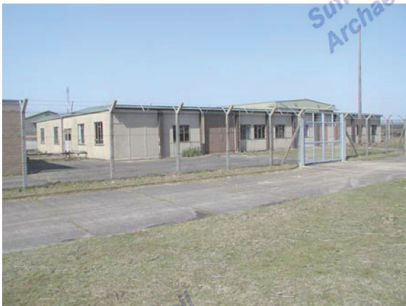
Building 214. View facing NW (P4260013)
