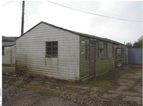
Building 14. View facing SW (P4280049)
