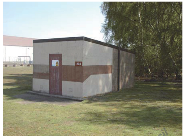
Building 234. View facing NE (P4260009)
