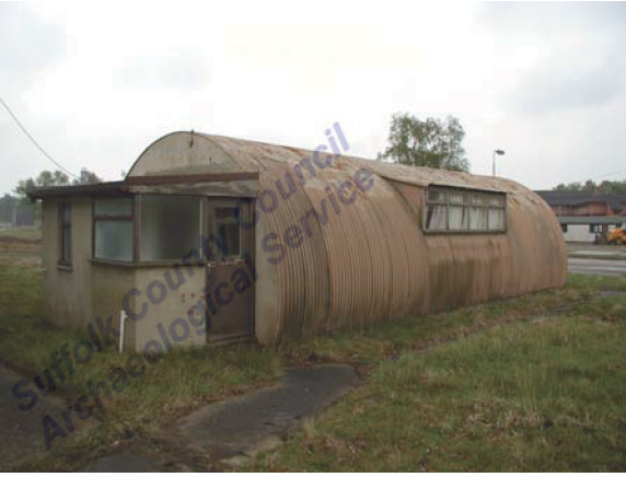
Building 21. View facing SW (P4280007)
