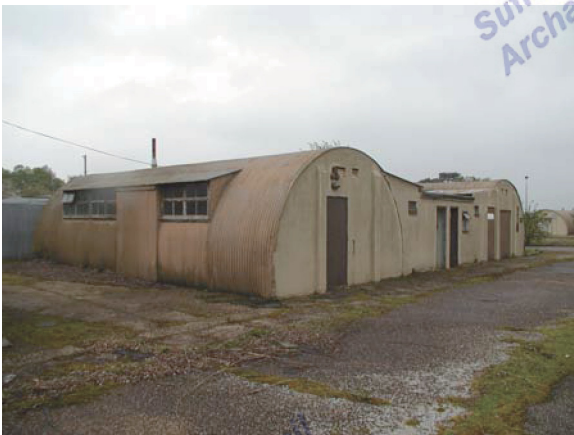
Building 13. View facing NW (P4280019)
