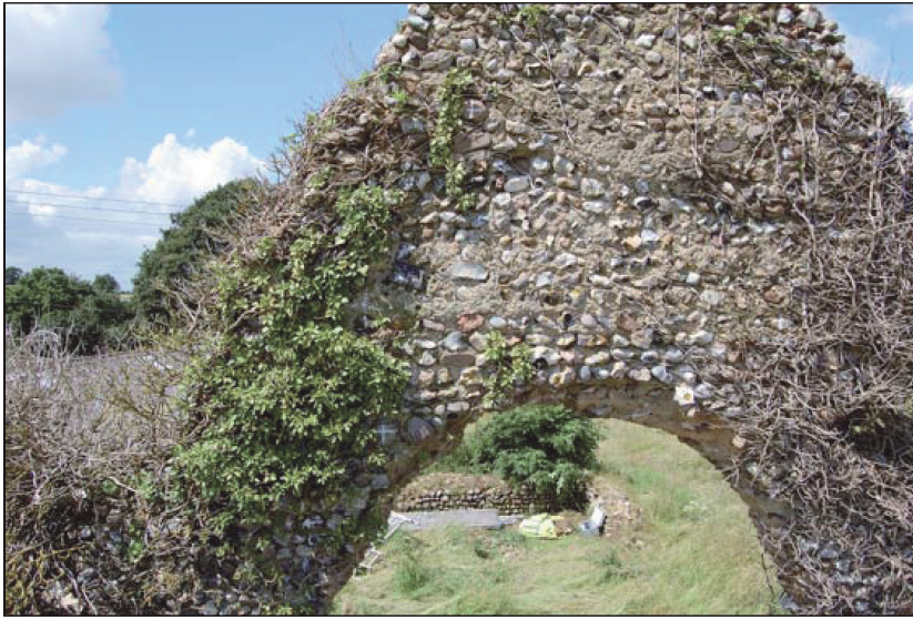
Figure 9. East elevation: Flush pointing and horizontal coursing
