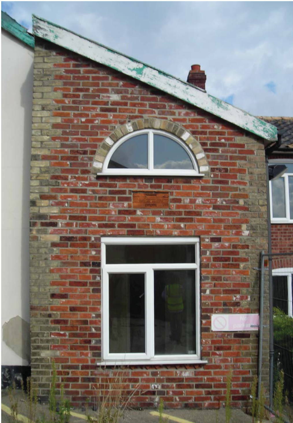
Fig. 15. Building D, viewed from the south
