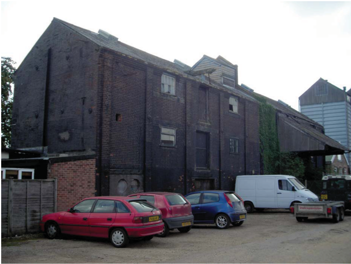
Fig. 9. Building A, viewed from the north-west
