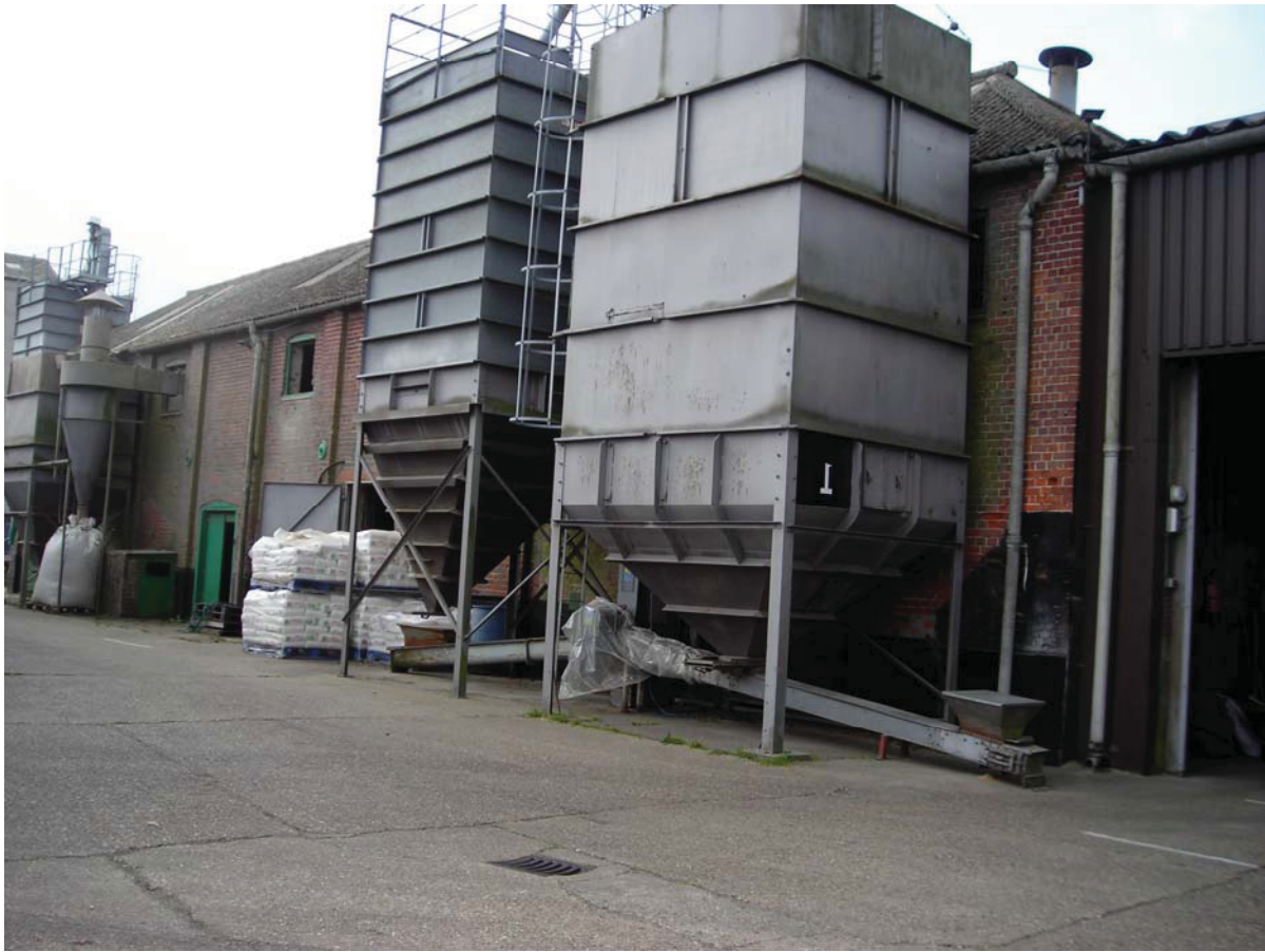
Fig. 13. Building C, viewed from the north-east
