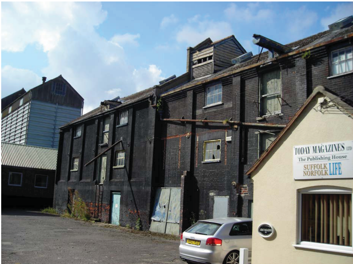
Fig. 10. Building A, viewed from the north-east
