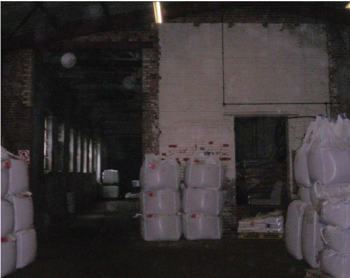
Fig. 12. Building B, viewed from the south
