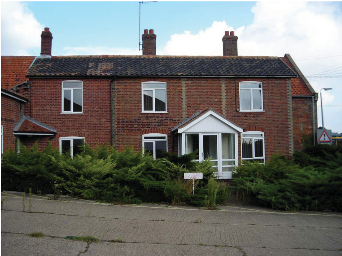
Fig. 14. Building E, viewed from the south
