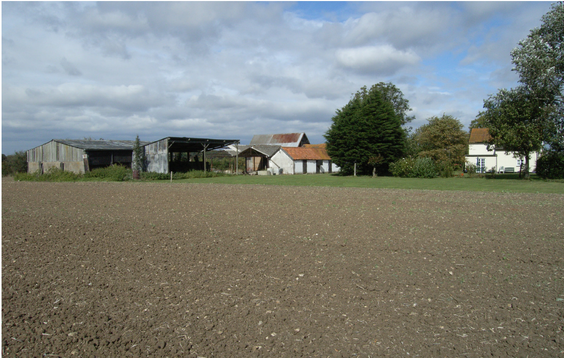
A2.1 General view of hilltop site from south showing farmhouse to right and redundant farm buildings to left
