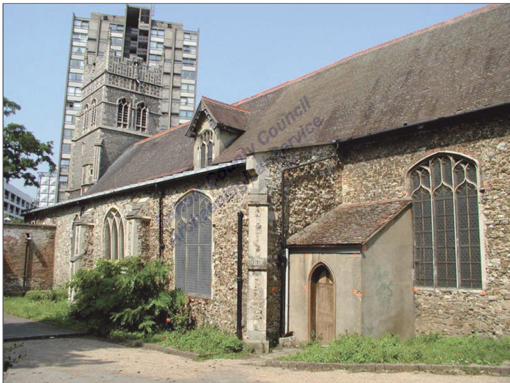
South Side of the Church
