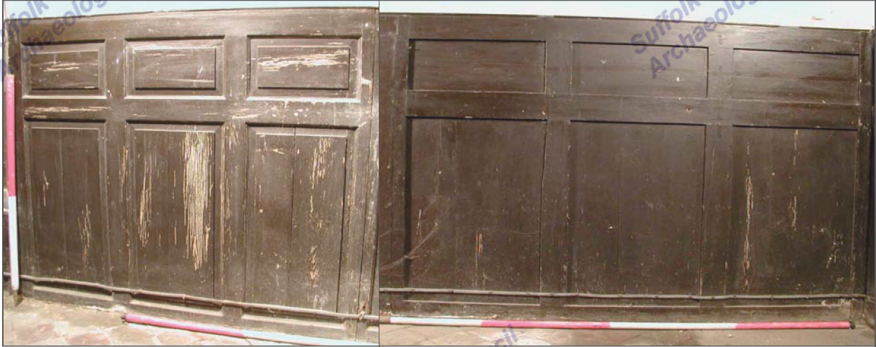
{A} N15; Fielded Panels Exposed
