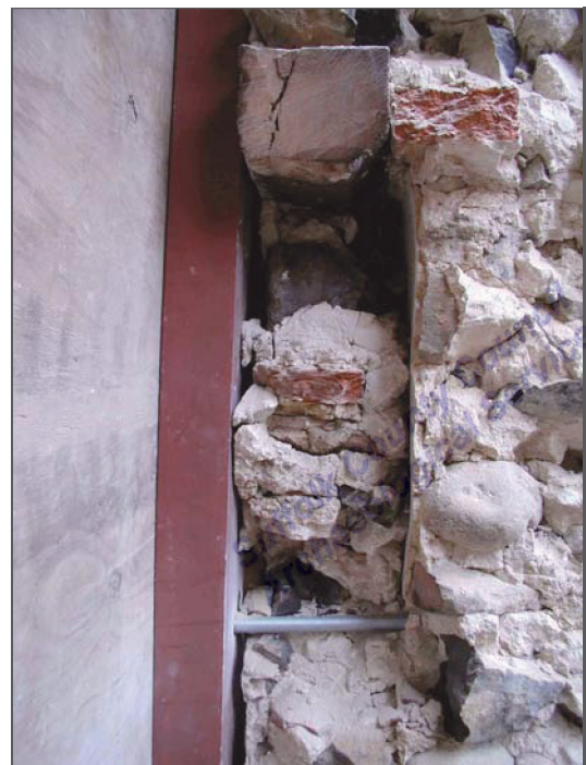
Plate 17: Detail of Filled Recess, South Aisle East Wall
