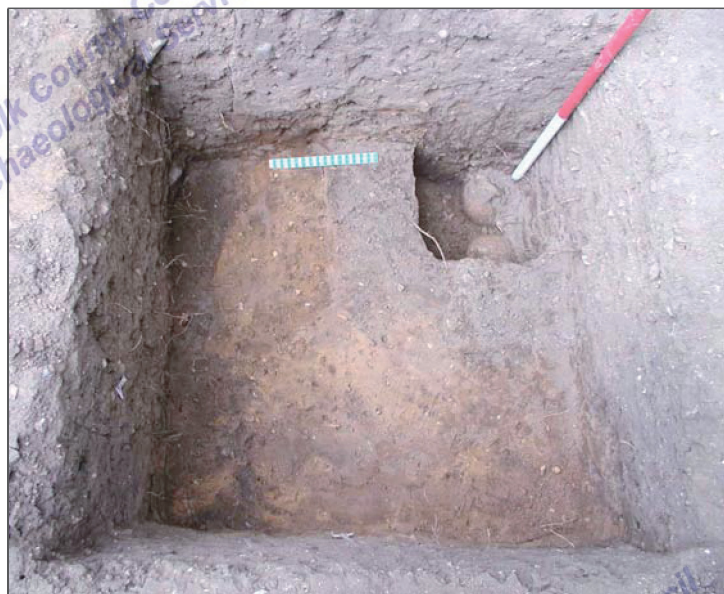
Plate 6: Excavated Footing Pad
