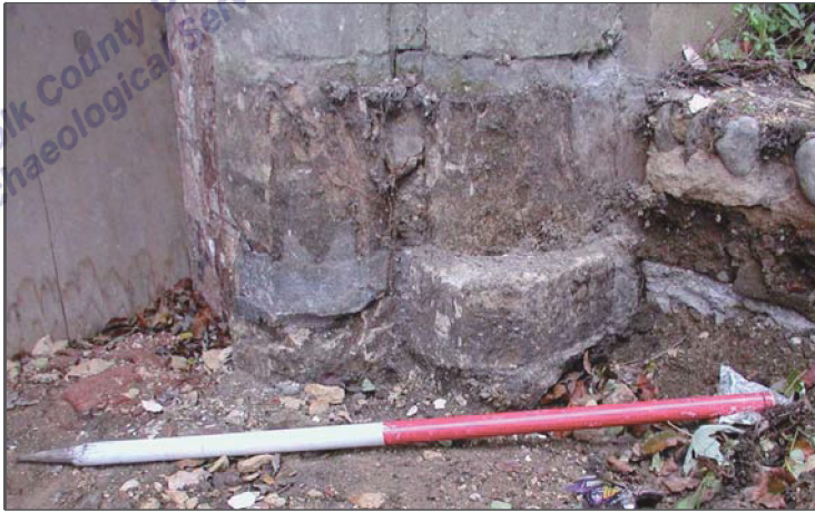
Plate 11: Detail of Moulding, West Side of North Doorway
