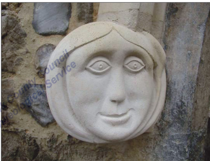
Plate 20: North Doorway; Replacement Label Stop
