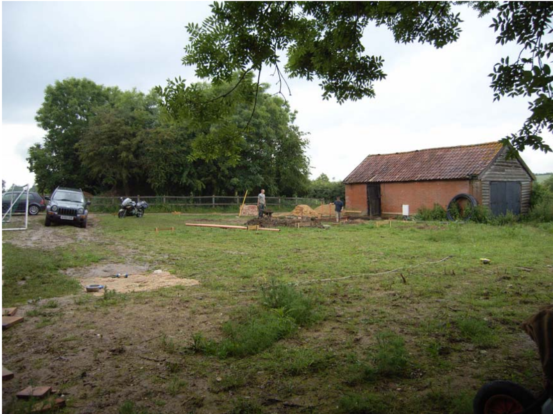
A2.1 General view of site from south across site of former brick sheds as shown on early plans. The brick kiln lies in the trees to the north.
