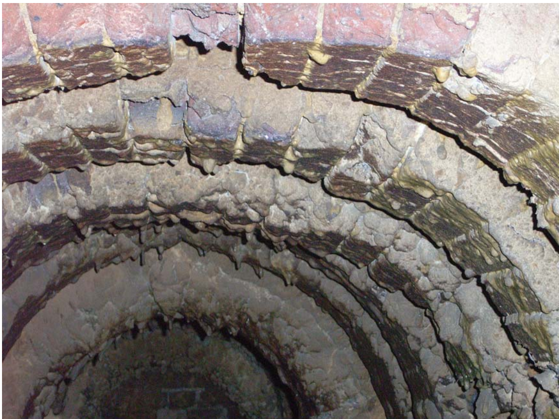
A2.6 Internal detail of one of the vaulted tunnels beneath the kiln, showing vitrification caused by intense heat (included for site context).
