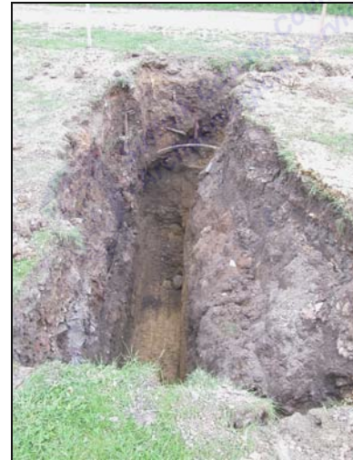
Plate III: footing showing area of deep excavation
