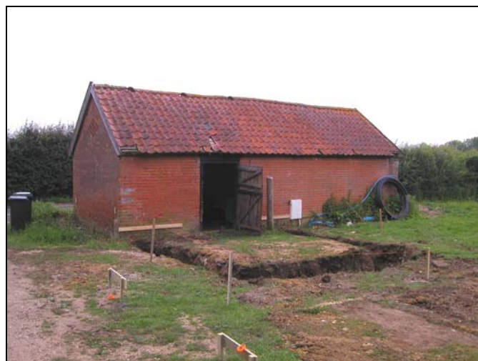
Plate I: Structure and footings (7-6-2007)
