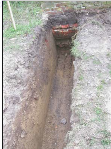
Plate II: footing adjacent existing structure
