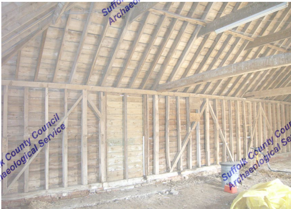
A2.4 Stable A. Interior of the eastern elevation showing a secondary blocked door and a small section of original cobbles. The machine-cut softwood framing is typical of the early-20 th century.
