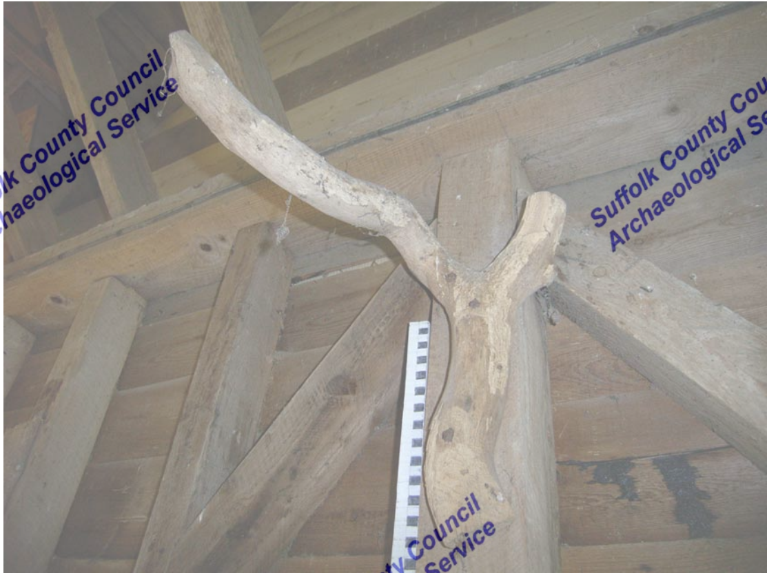
A2.5 Stable A. Detail of the southernmost of two bentwood harness hooks nailed to the western wall at its northern end.
