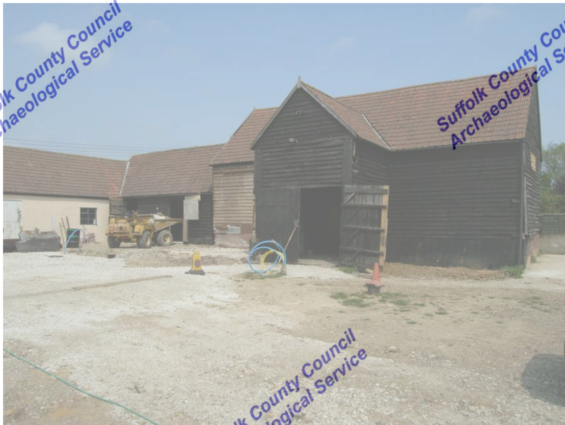
A2.1 The eastern side of the yard from the south-west, showing from left-to-right the 20 th century buildings marked on the Block Plan as Shed D, Stable A and Barn B.
