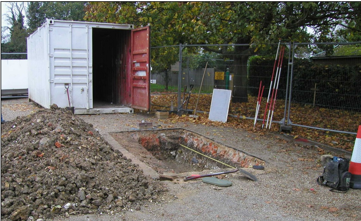
Plate II: General view, looking northwest
