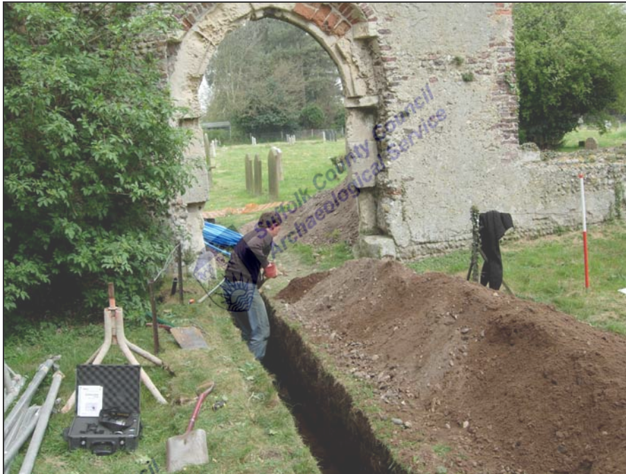
Excavation in progress
