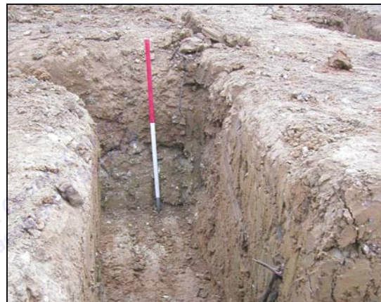
Plate II: Excavated Footing
