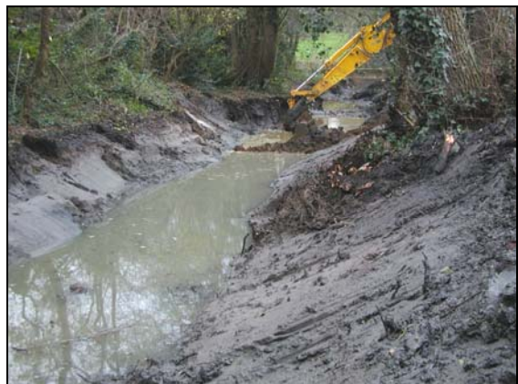
Plate VIII: desilting the moat
