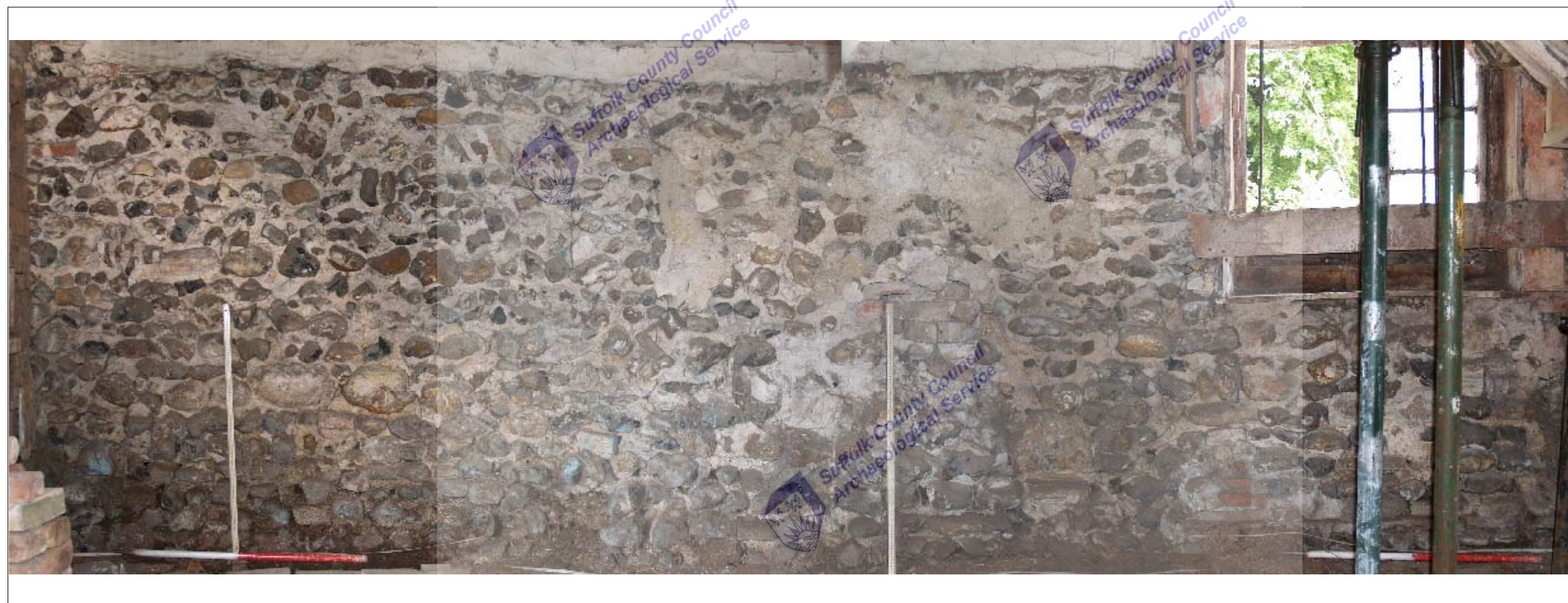
Plate 2: Batemans Barn, North Wall, Internal Elevation (East End)
