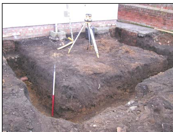
Plate II: Excavated Footings for No. 118
