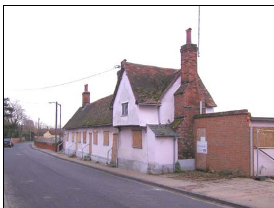
Plate I: General View from Benton Street view looking south
