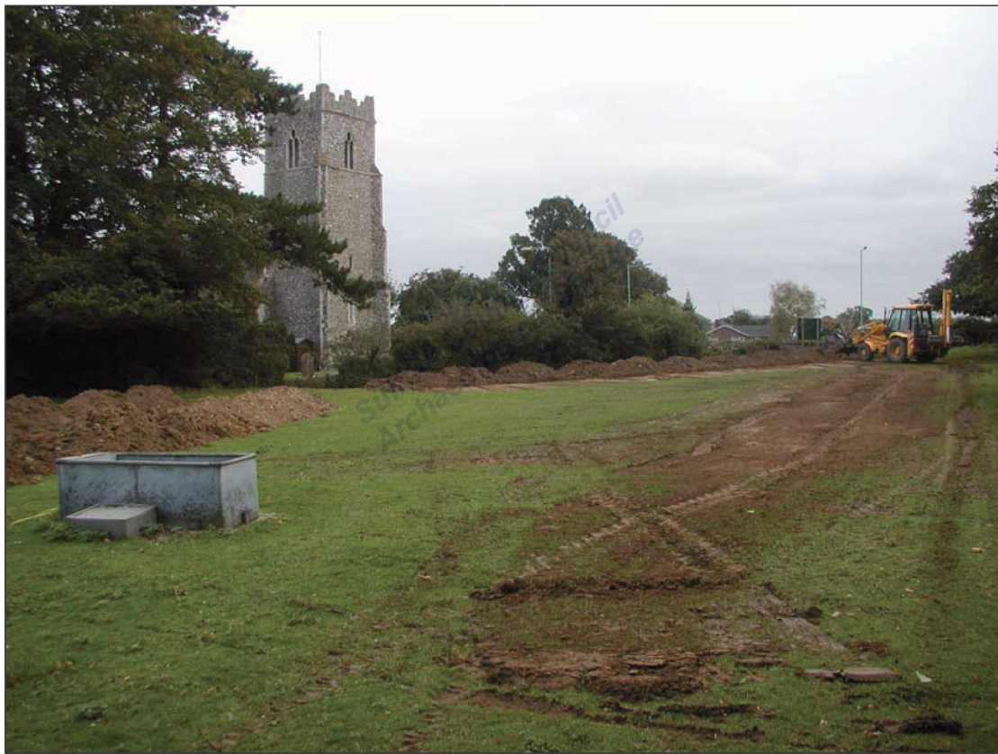
Figure 1: View of the trenched area looking south towards St Peter's Church
