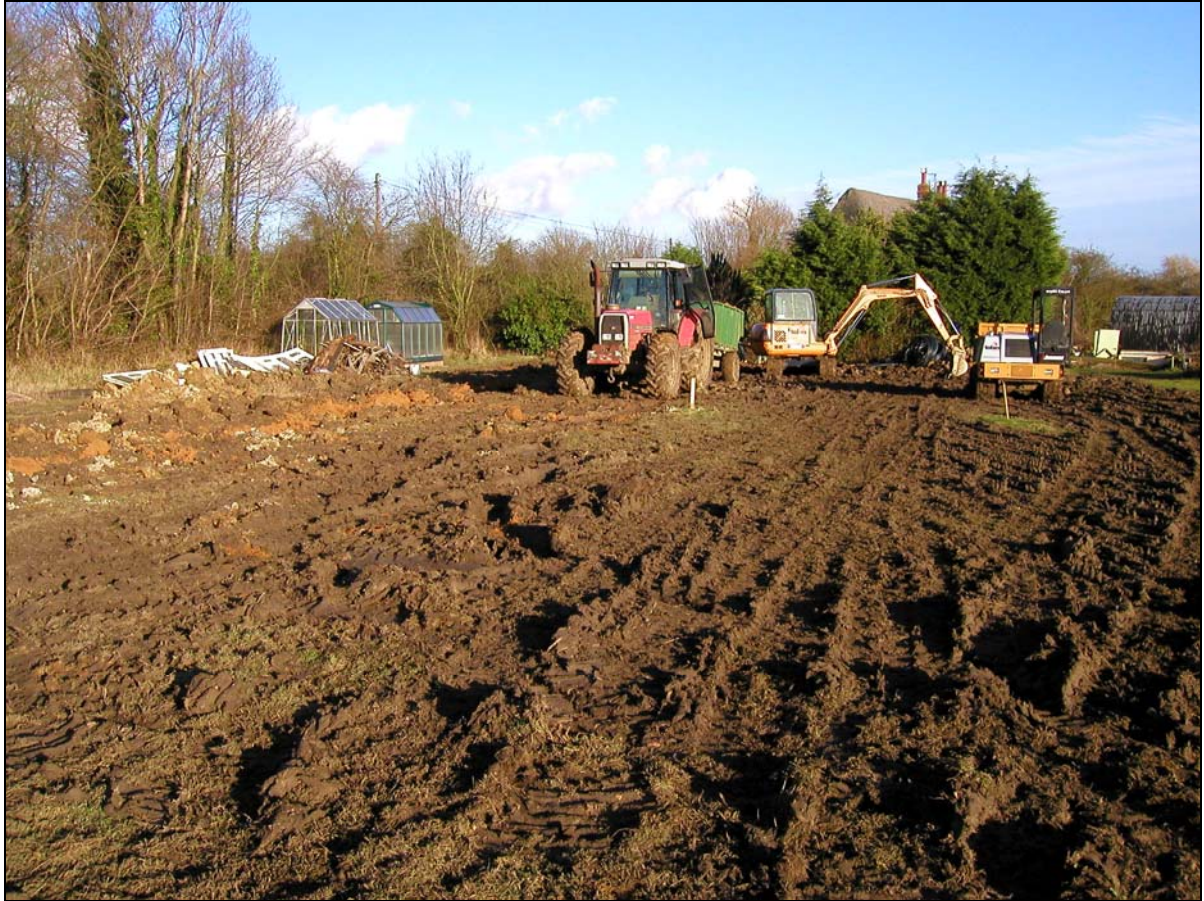
Work Underway, view looking NE (24 th January 2008)
