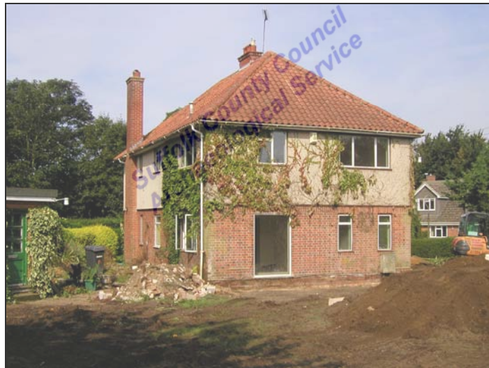
Plate I: Castle Orchard House prior to extension (view facing west)
