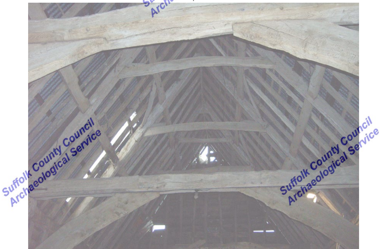
A2.6 Roof structure showing all four original tie-beam braces from west
