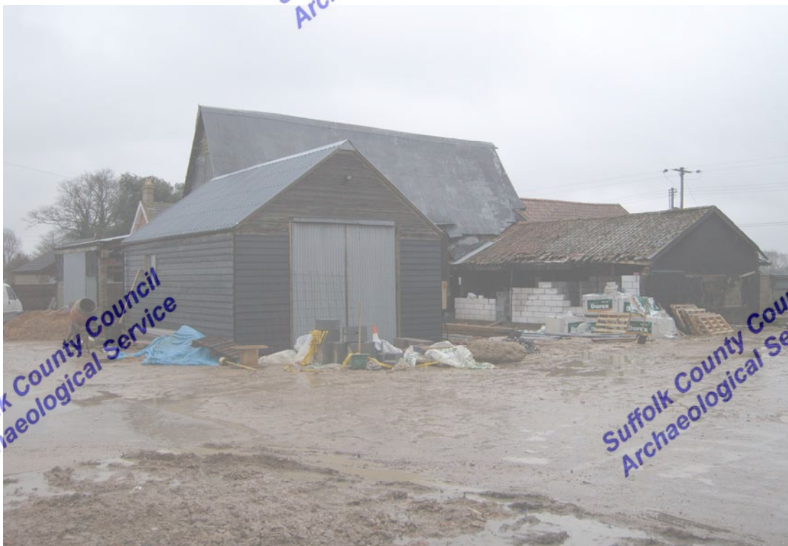
A2.2 General view of site from west showing barn behind Yard A with Shed (10) in foreground
