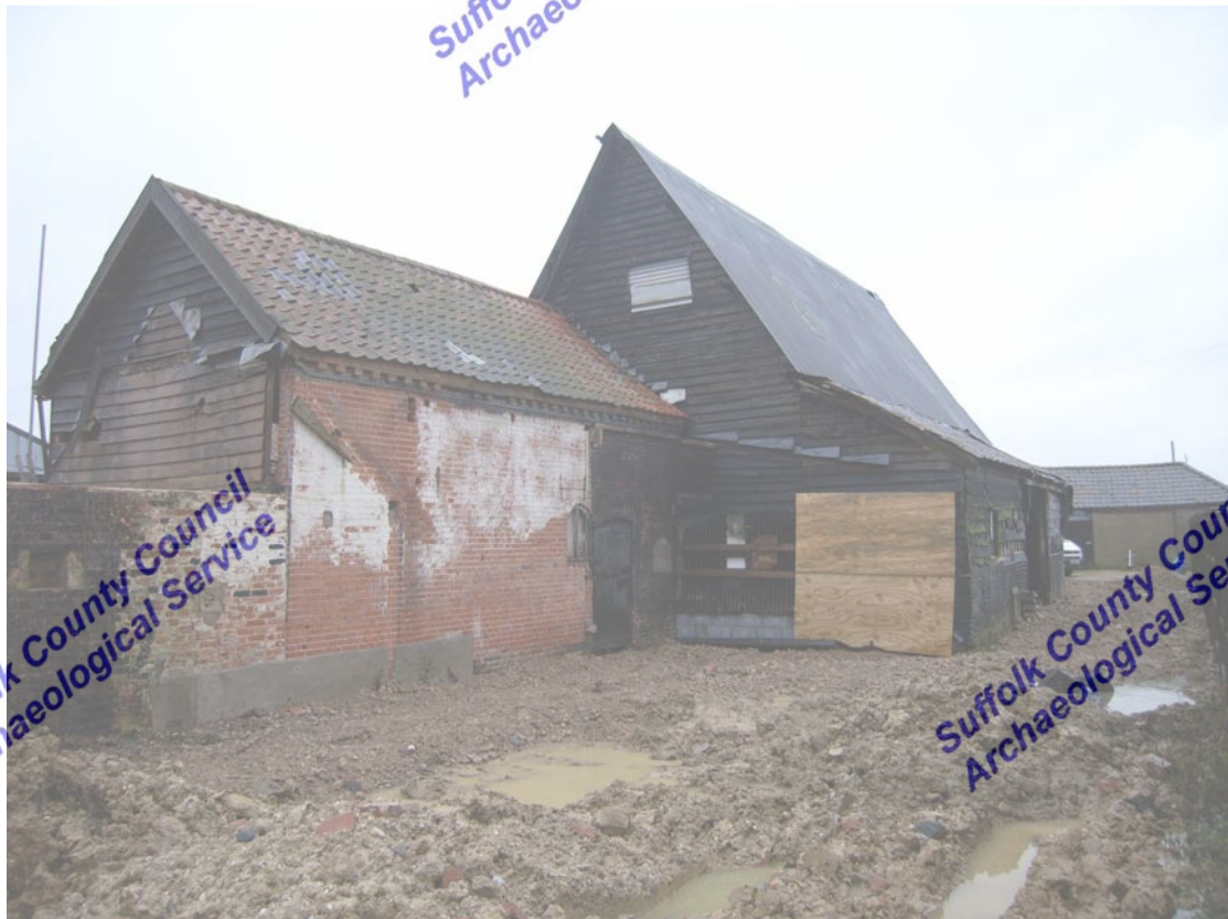
A2.4 Exterior from east showing Stable (5) to left with barn in rear. Note scar of demolished building which projected to north-east
