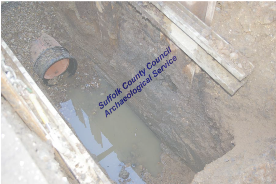
Figure 3. General view of the sewer trench, looking southeast
