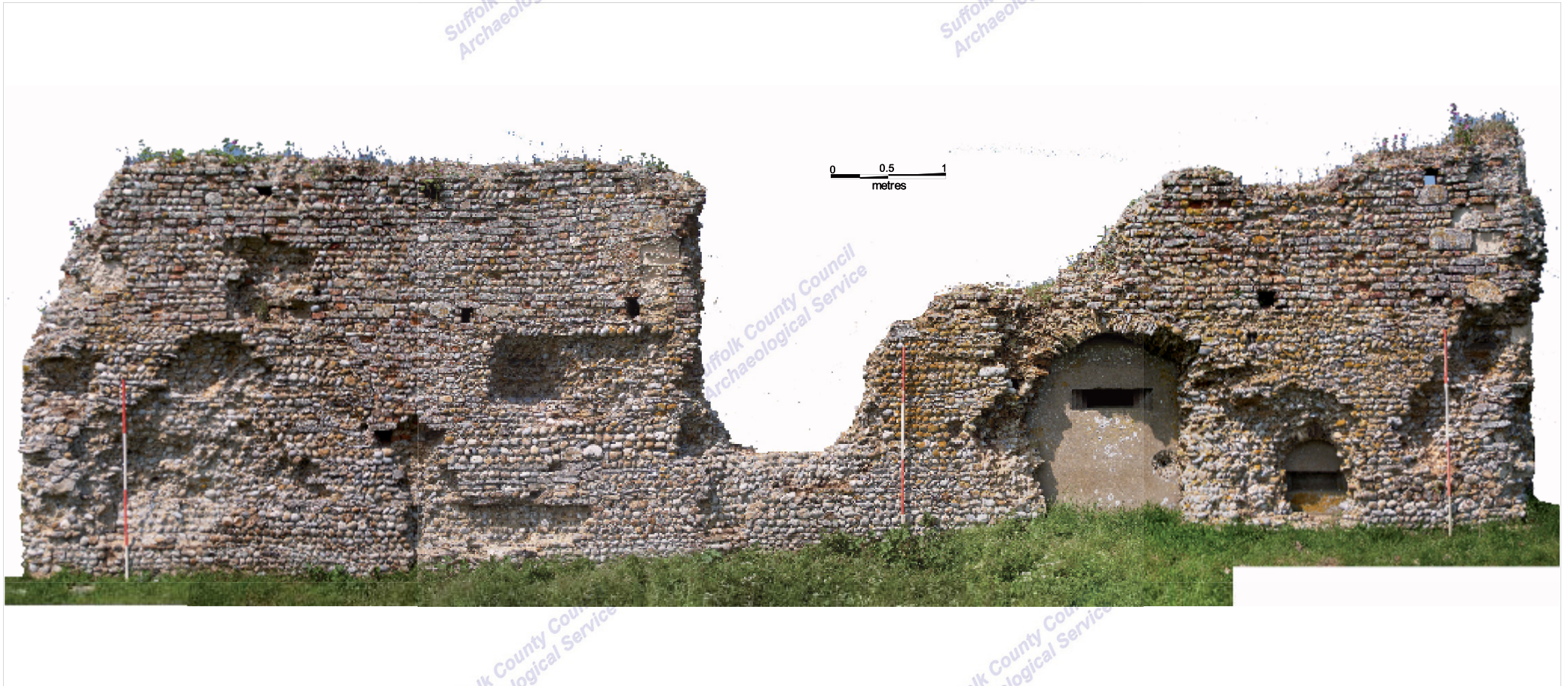
Plate. 6 South exterior elevation, composite photograph
