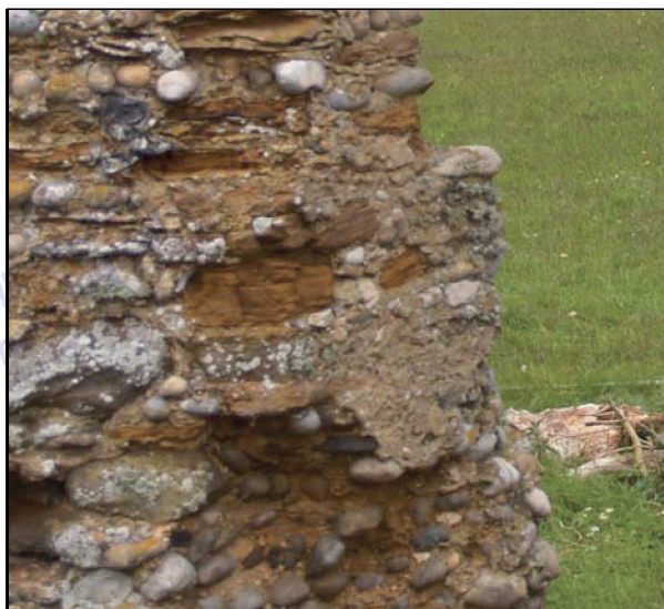
Plate 18 Detail surviving splay in window 0082
