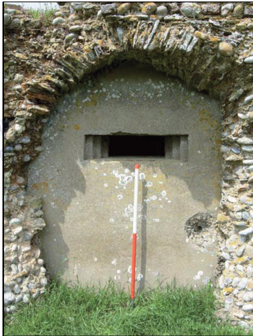
Plate 23 Detail of doorway 0085
