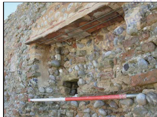
Plate 38 Drip course in south wall
