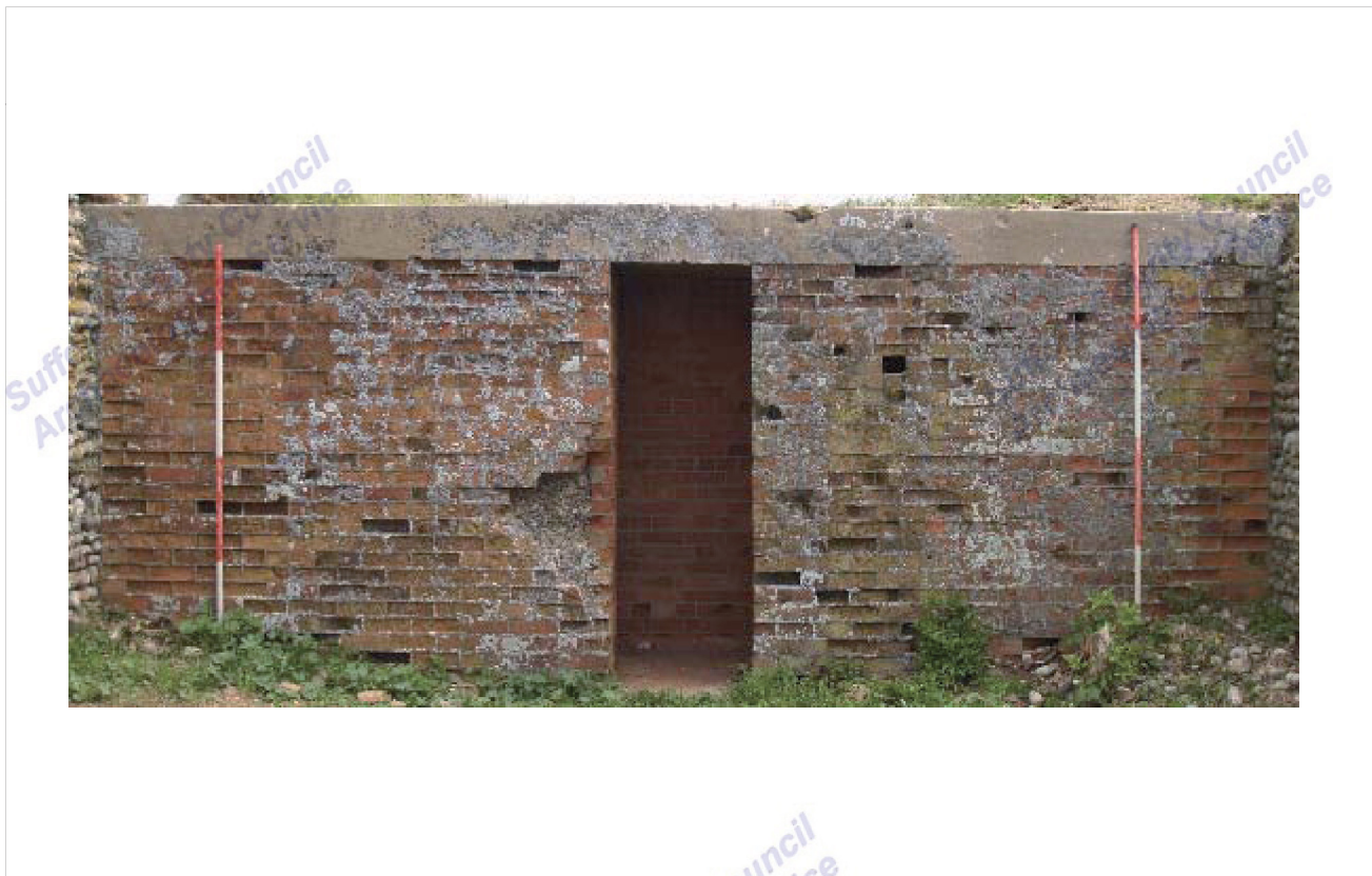
Plate 11 Pillbox west exterior wall, composite photograph
