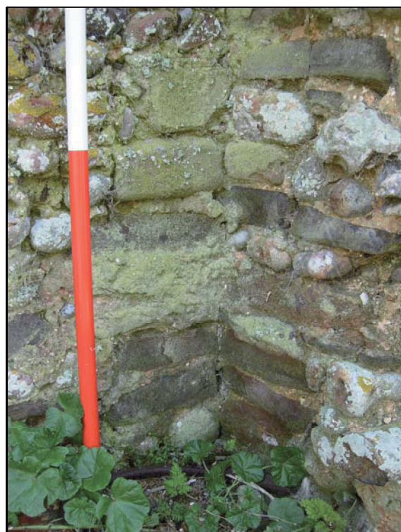
Plate 21 Detail of south-west internal corner
