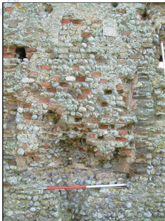
Plate 20 Blocked window 0083, internal view
