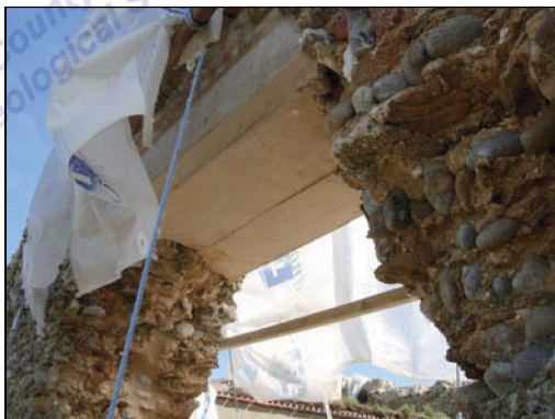
Plate 37 Concrete lintel in 0082
