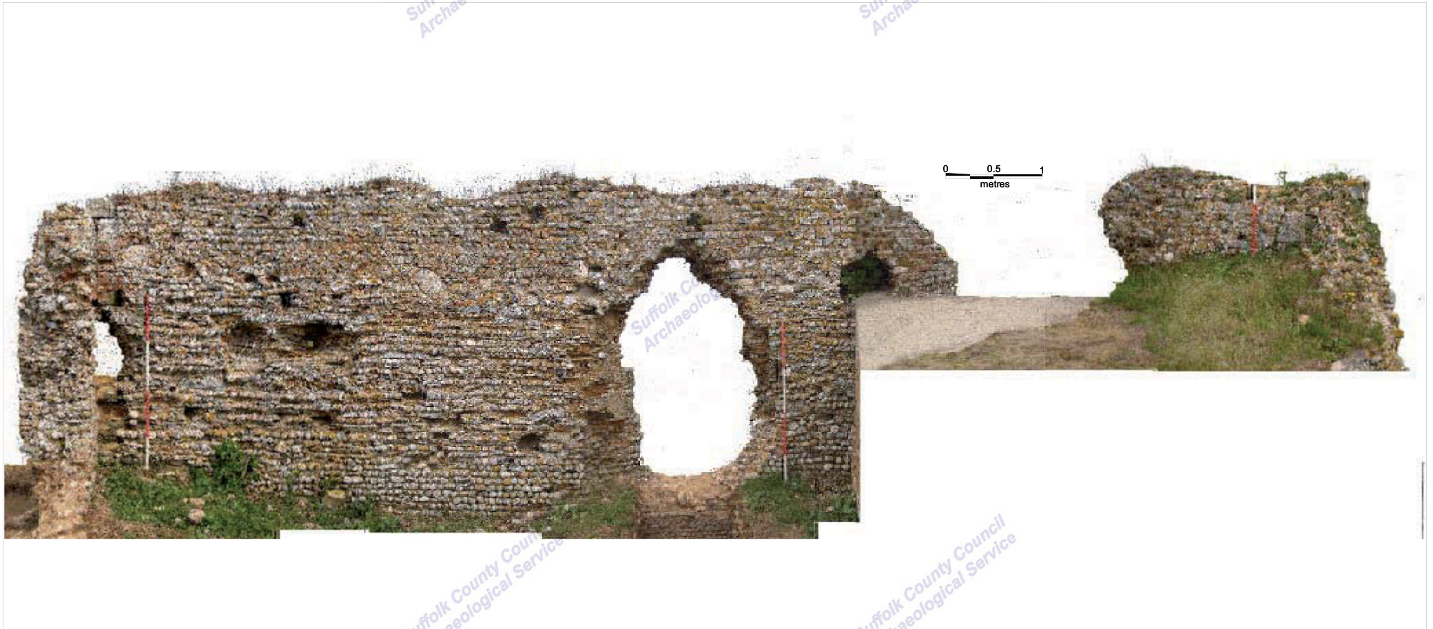
Plate 5 North interior elevation, composite photograph
