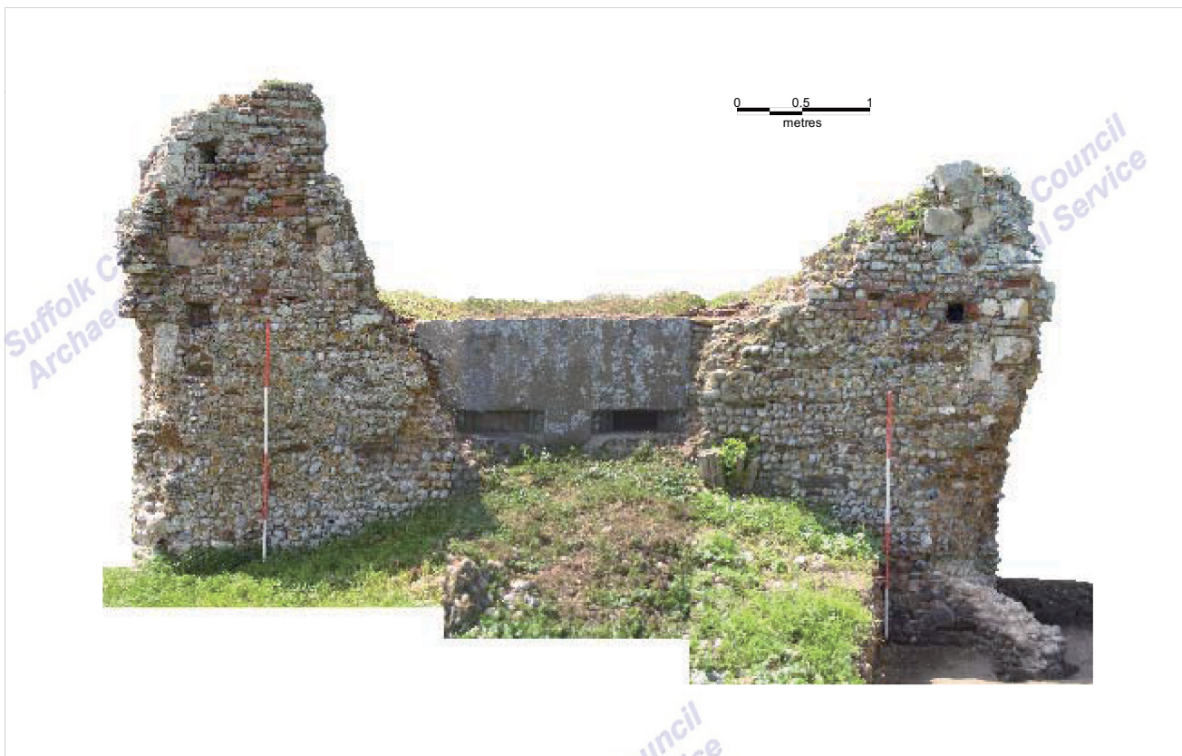
Plate 8 East exterior elevation, composite photograph
