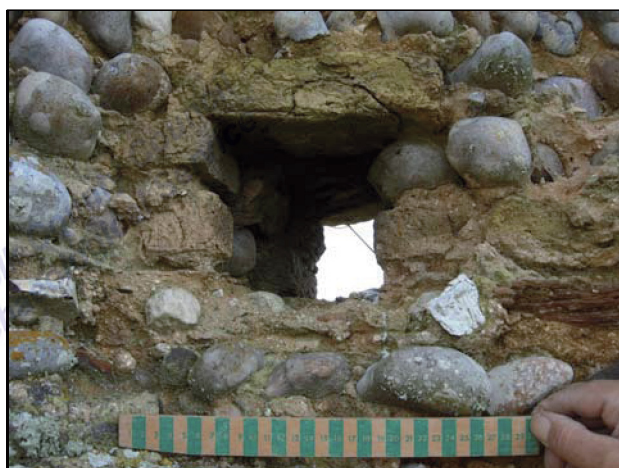
Plate 30 Detail of brick lining in putlock hole 0097
