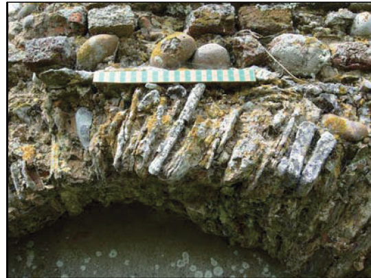
Plate 24 Detail of doorway arch 0085 of hard ferruginous sandstone lain face to face radially around the top of the feature (Plate 24). This pattern may have once continued down the jambs, but all facing at this juncture had been compromised.
