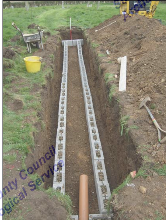
Plate 4 Trench Arch Drain
