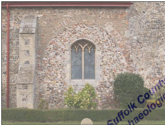
Plate 3 Detail of blocked chapel arch
