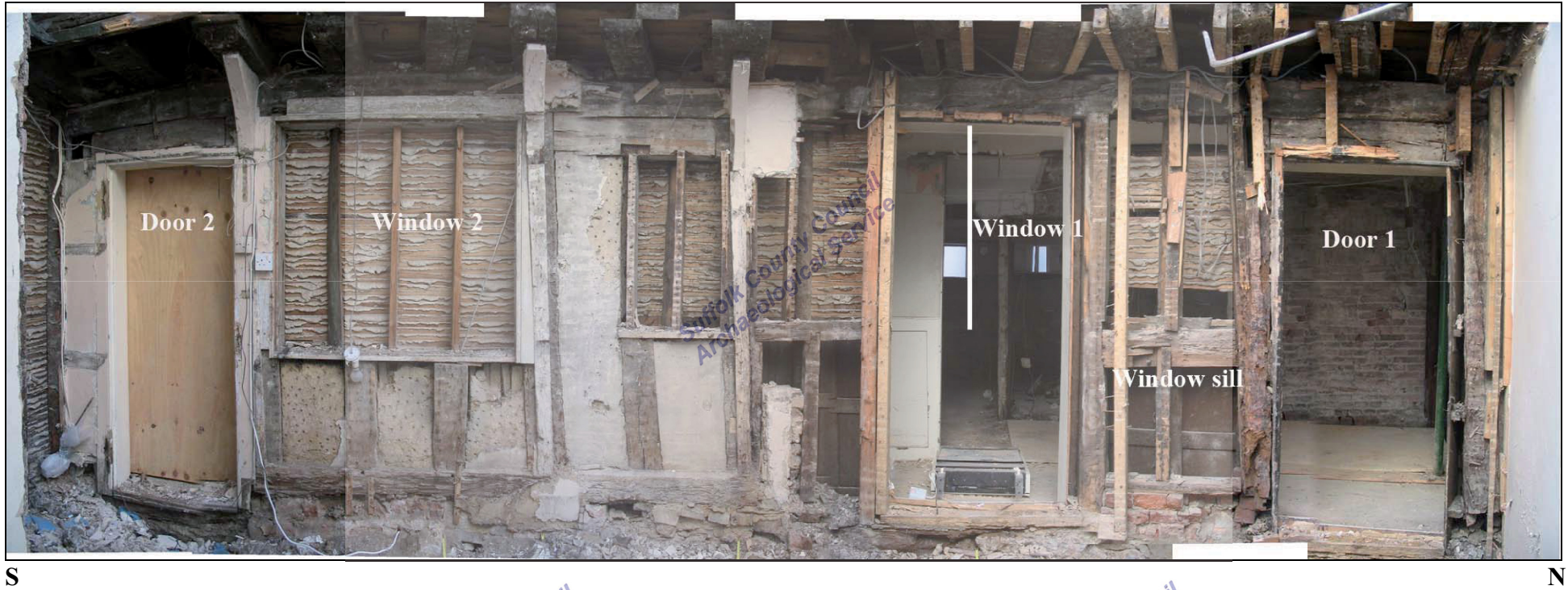
Figure 6. East face of timber-framed building (photographic mosaic from architect's photographs).
