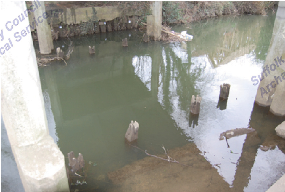
Figure 2. Timber piles of the 1790's bridge below the present concrete bridge (built 1922)
