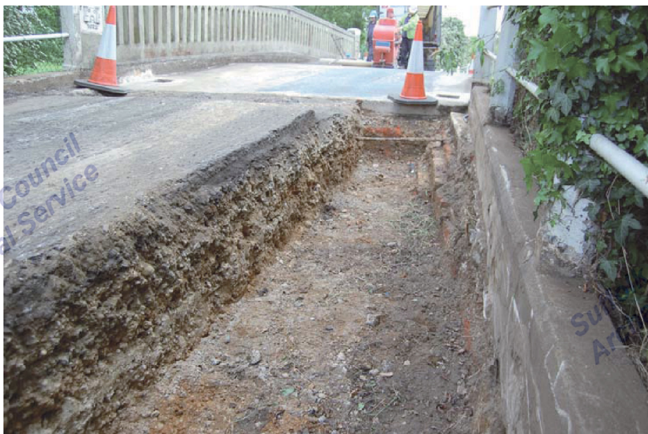
Figure 9. Trench showing road make-up and south wall of the west abutment
