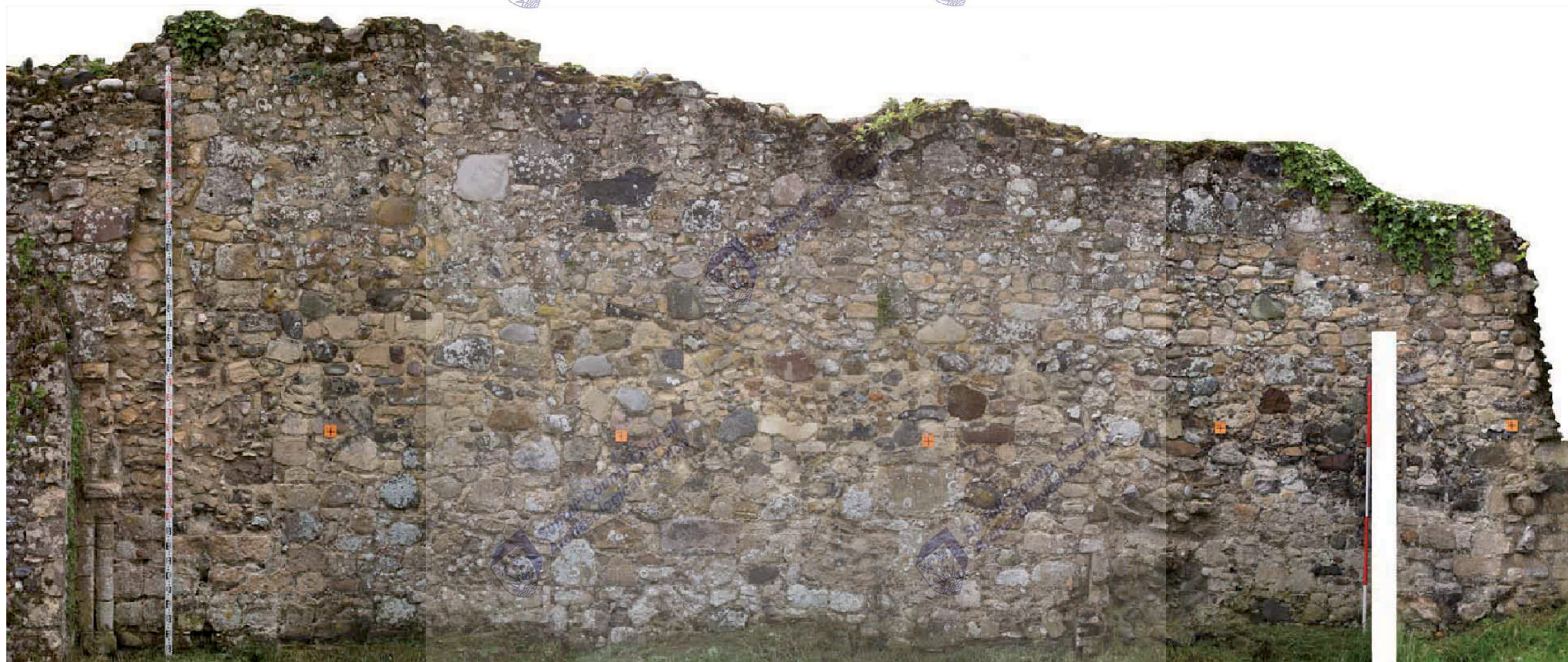
Plate 10 South wall of Nave/Hall & Chancel (internal); composite photograph (scale c.1:50)
