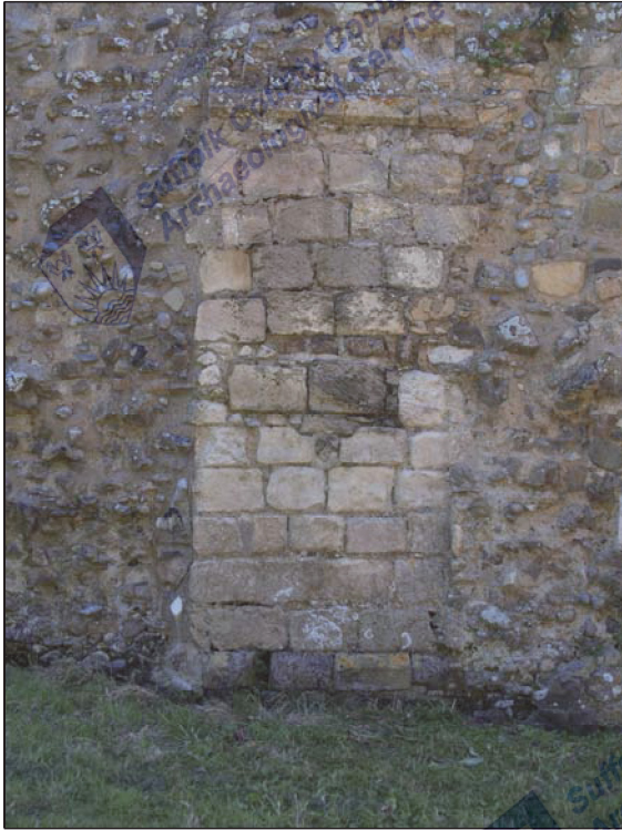
Plate 2 Apse ashlar fabric 0034 with putlock hole 0035
