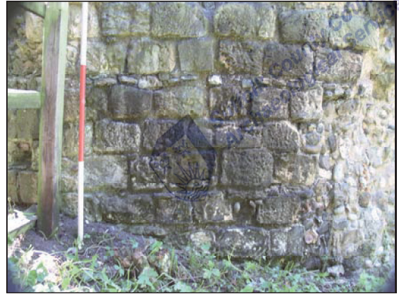
Plate 3 Ashlar fabric 0079 with galleting & putlock hole 0085
