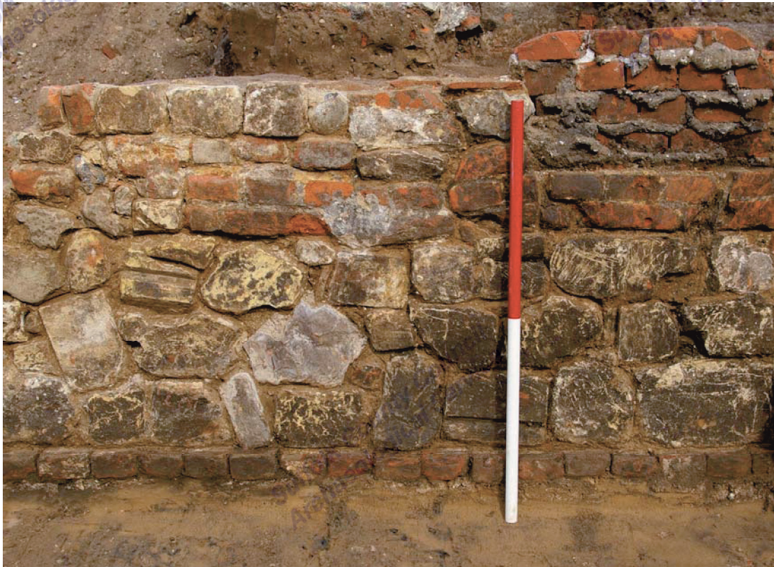
Figure 7. Part of the northeast wall of Building 1, displaying the extensive re-use of architectural mouldings. Note that the brick masonry bonded with grey mortar above and to the right of the photographic scale is part of a later structure (1m scale)
