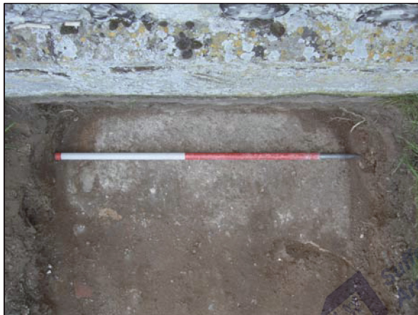
Plate 6 Stepped out external footing
