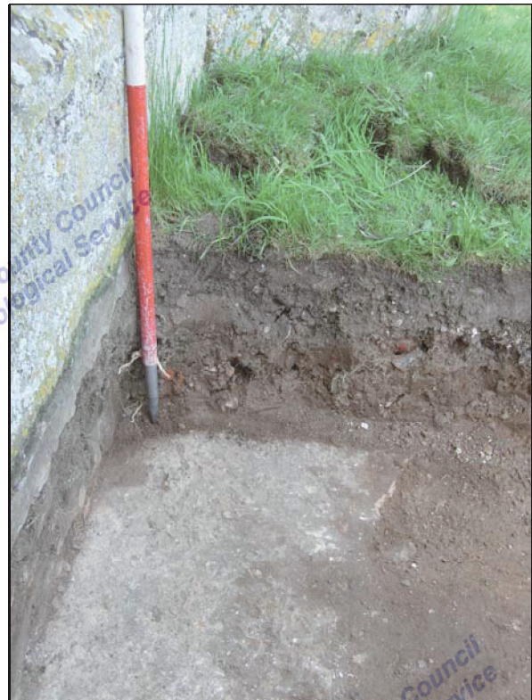
Plate 7 Stepped out external footing & overburden
