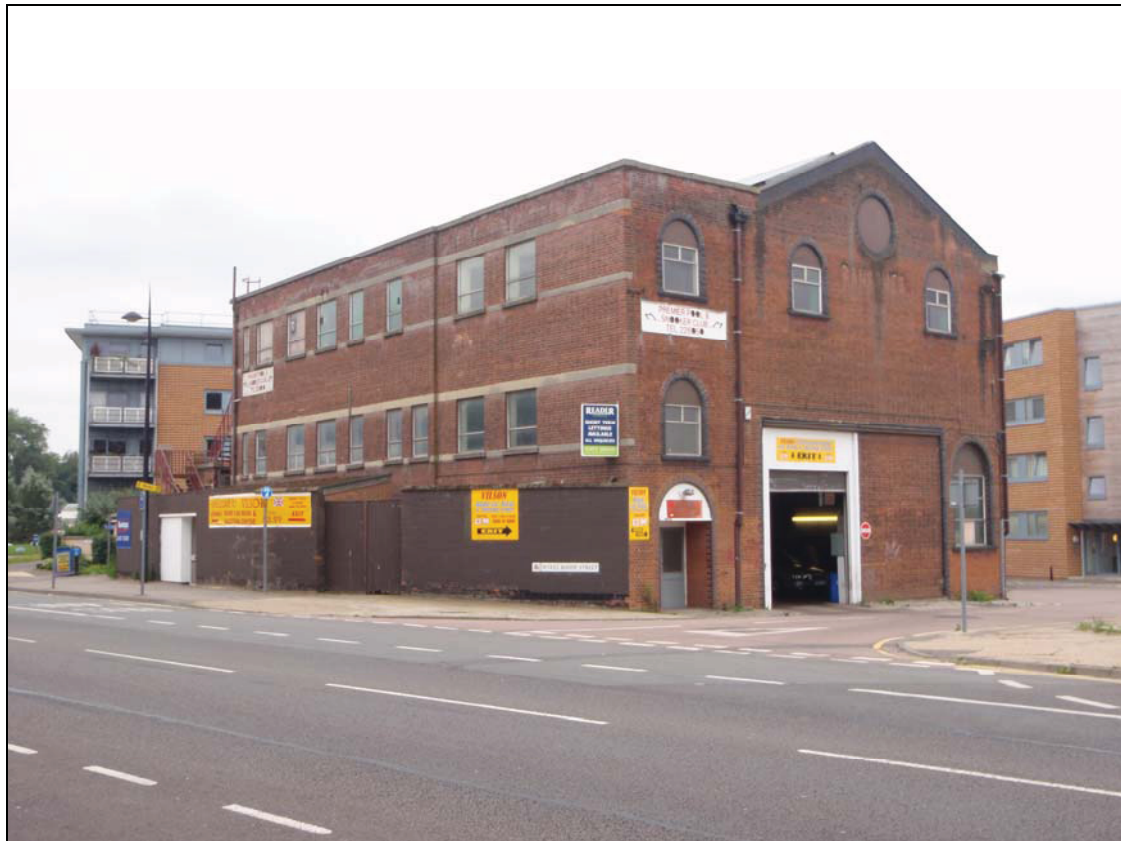
Island House, 28-8-2008, view looking south
