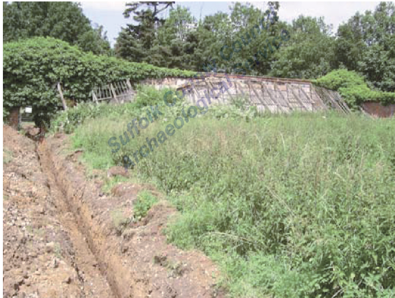
Figure 14. Service trench through walled garden.
