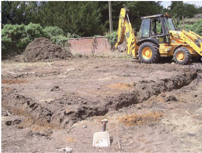
Figure 13. Garage 3 during excavation
