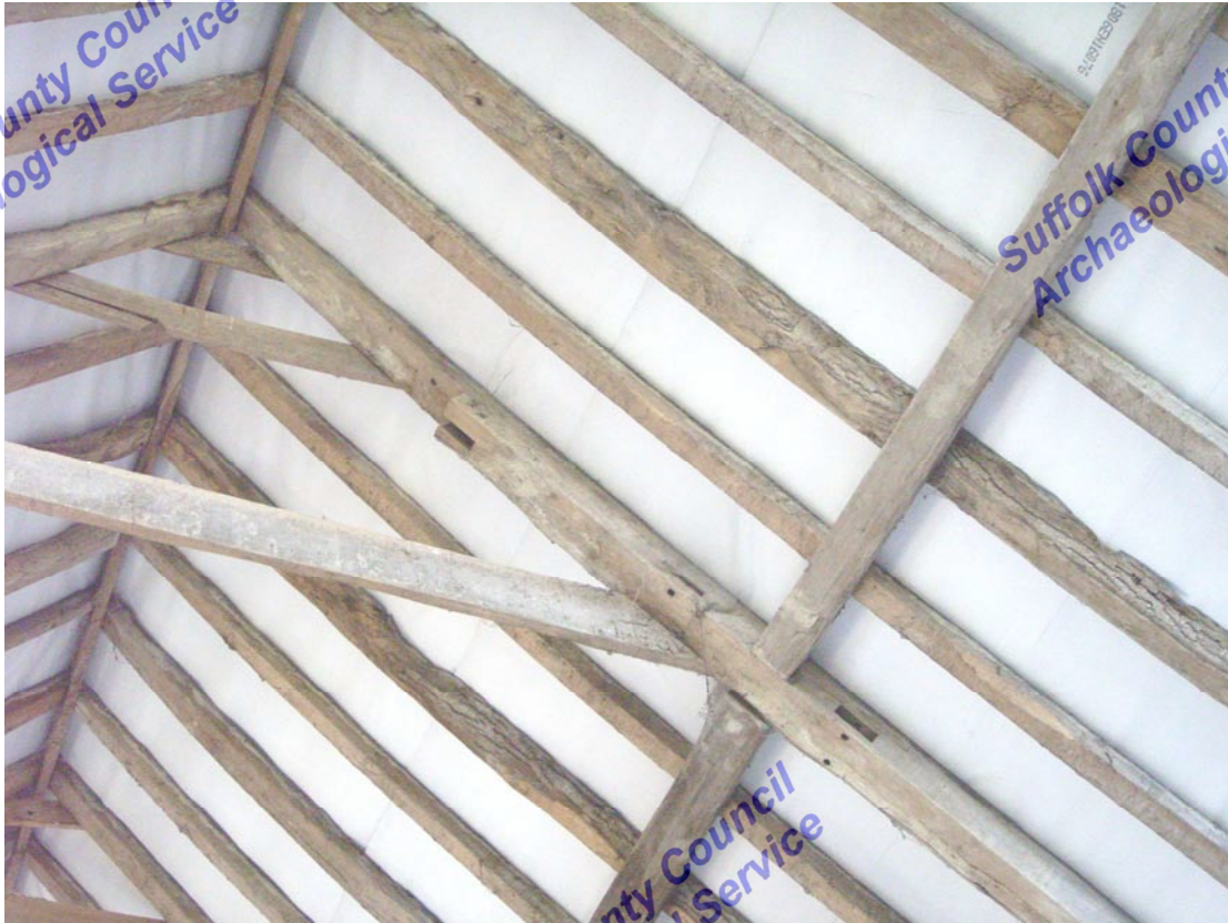
A2.5 Detail of 19 th century butt-purlin roof structure showing re-used 17 th century principal rafter with empty mortises for an upper tier of clasped purlins with wind-braces and a lower tier of butt-purlins
