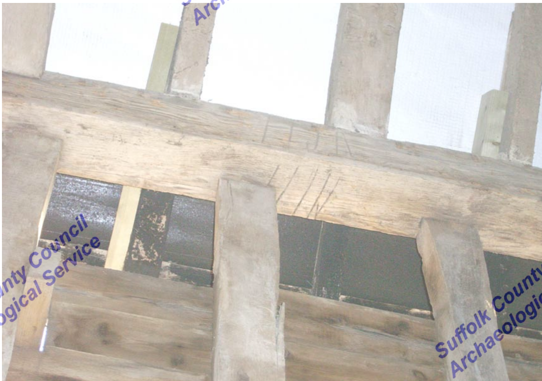
A2.6 One of several Baltic timber marks on the 19 th century pine roof-plates in both elevations
