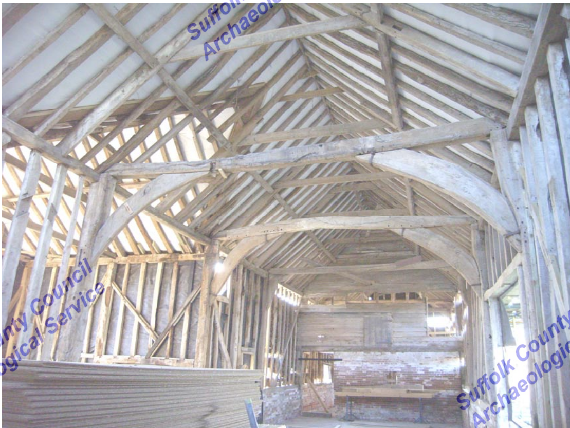
A2.4 General view of barn interior from east showing re-used tie-beam arch-braces flanking bay F with porch to left and brick and boarded partition to stable in rear.
