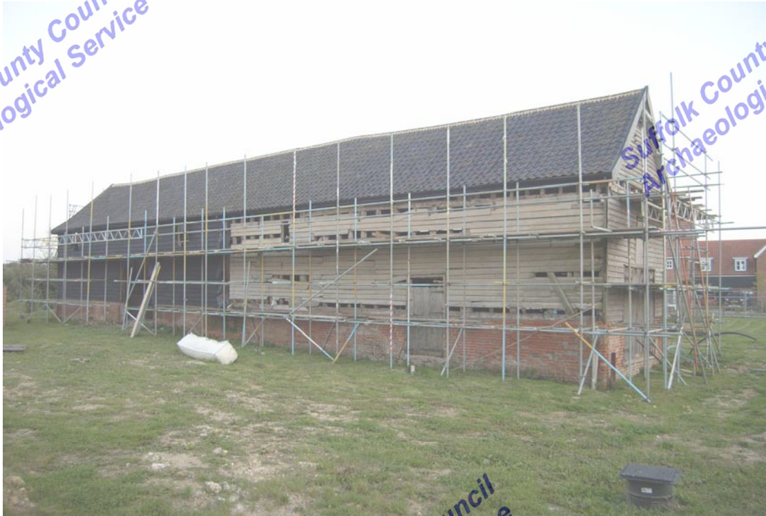
A2.3 Northern external elevation from north-west showing old whitewashed weatherboarding to right (formerly enclosed by a recently demolished shed) with recently renewed stained boarding to left
