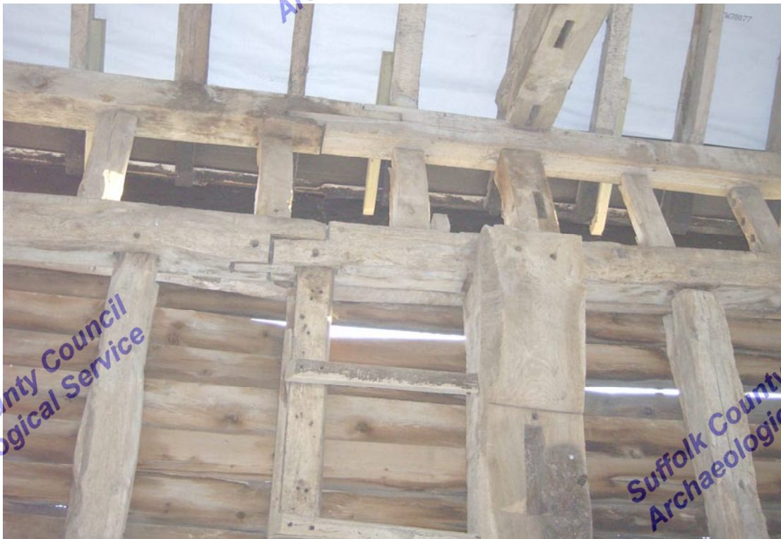
A2. 10 Detail of jowled northern storey post between bays A (left) & B showing 19 th century roof-plate with edge-halved scarf joint and mortise for original ceiling joist
