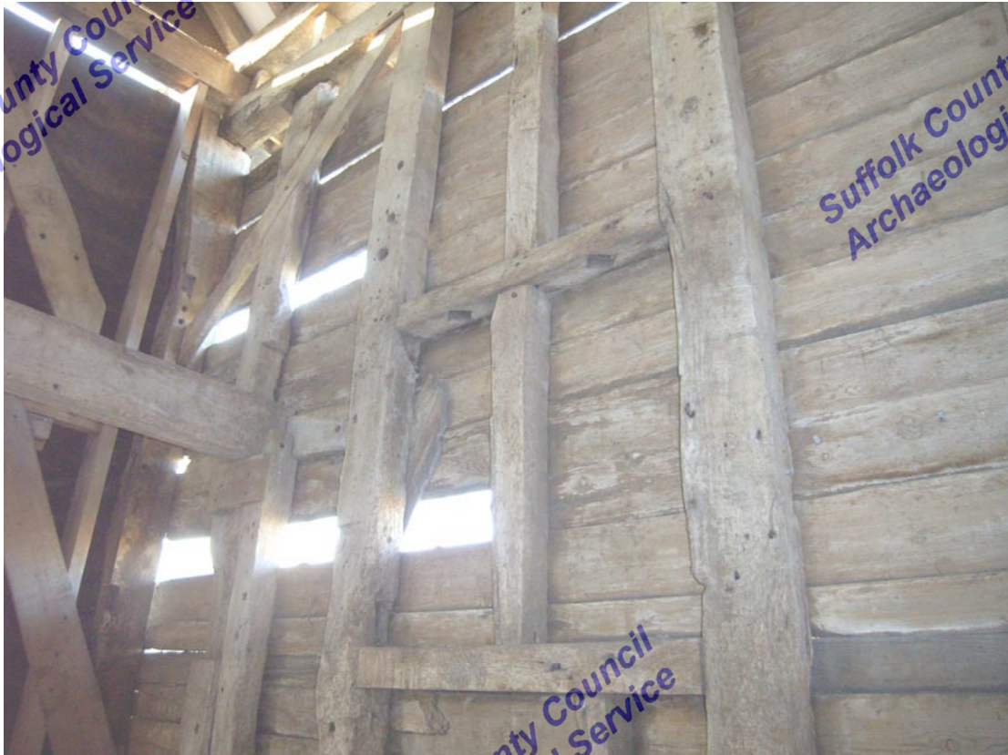
A2. 9 Lintel of 17 th century stable window lintel with empty mortises for three diamond mullions in bay A with original internal wall brace top-left (the empty sill mortises are visible above the present secondary sill)
