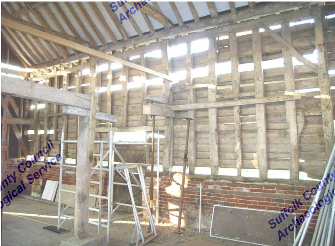
A2.8 Northern internal elevation of stable from south-east, showing bays A-C from left to right. The entire structure raised on a brick plinth and provided with a new, higher roof-plate
