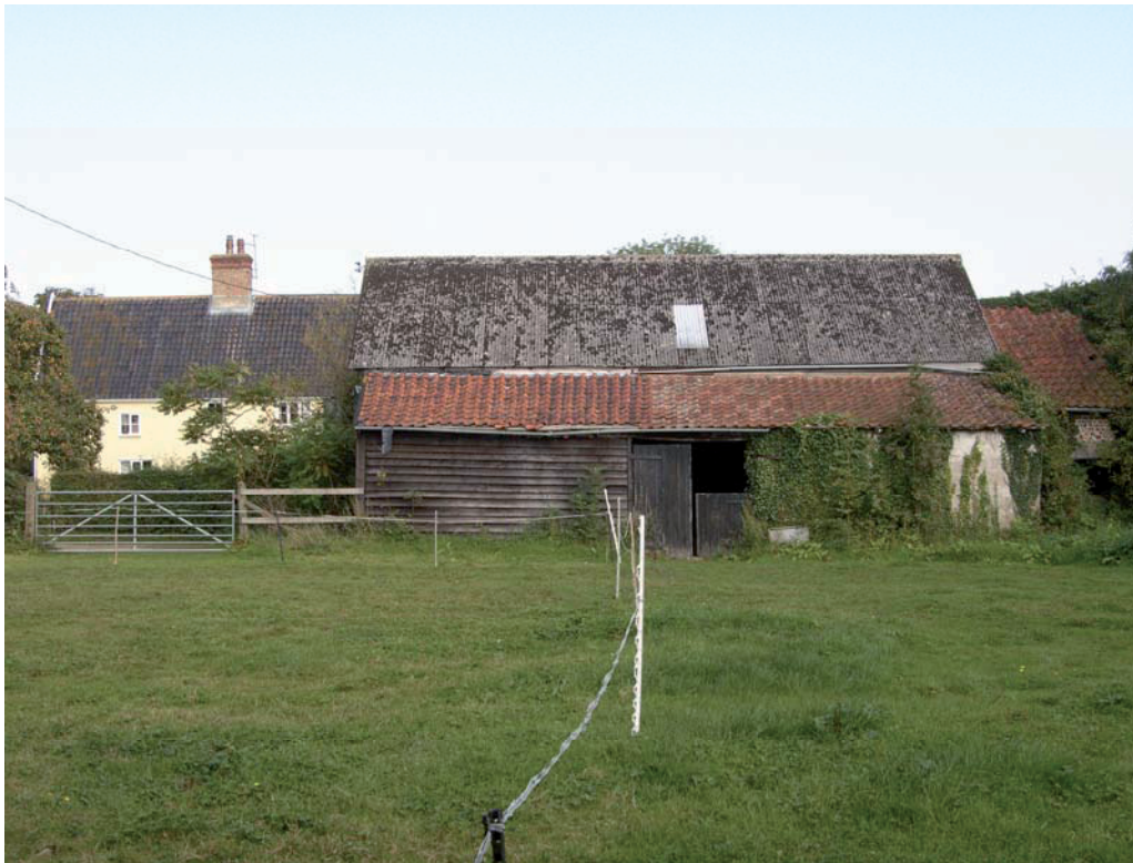
A2.1 General view of site from west showing barn (1) in centre with later lean-to in foreground; brick stable (2) to right and listed farmhouse (4) to left
