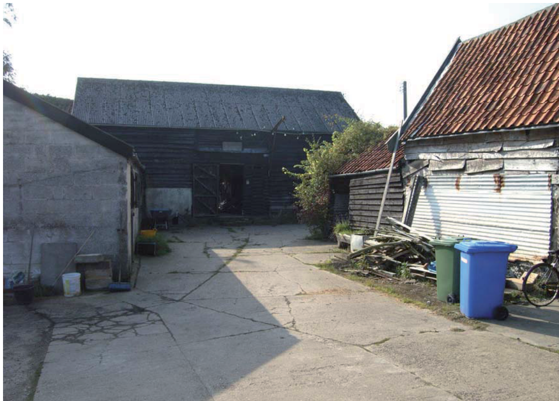
A2.2 Exterior of barn (centre) from yard to east showing timber-framed stable (3) to right & modern block-work stable to left
