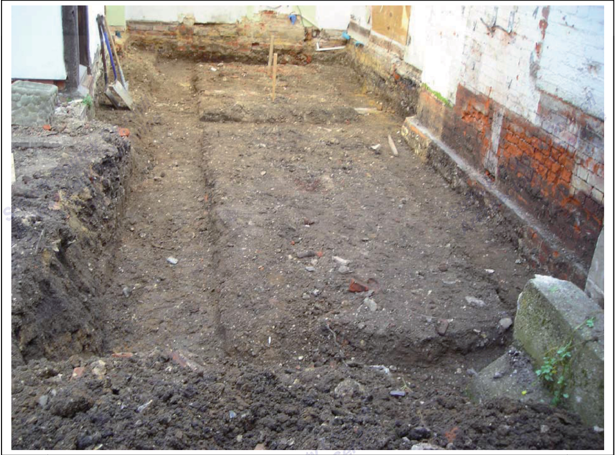
Plate 1. View of excavated extension footprint, looking south
