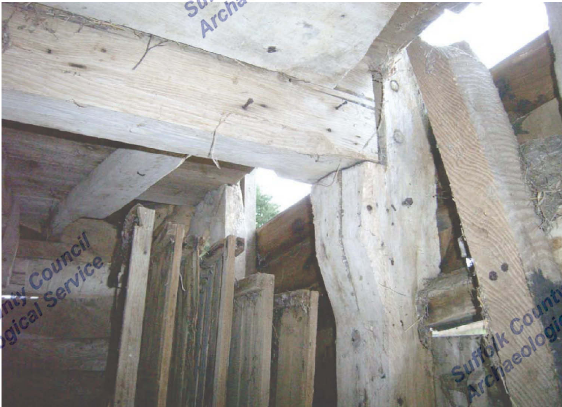
A2.18 Barn. Detail of stable ceiling showing chamfered binding joist and corbel block to western post
