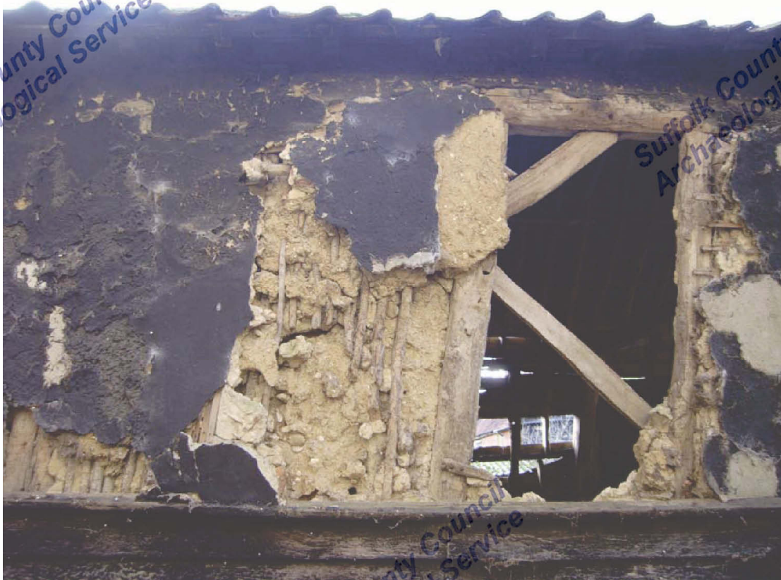
A2.13 Barn. Detail of tarred external wattle-and-daub to eastern elevation
