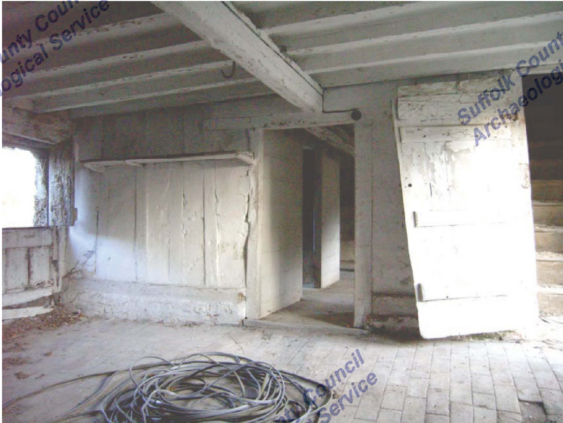
A2.7 Bakehouse. Interior from west showing timber-framed partition with central door to eastern storeroom, rear external door to left and stair door to right
