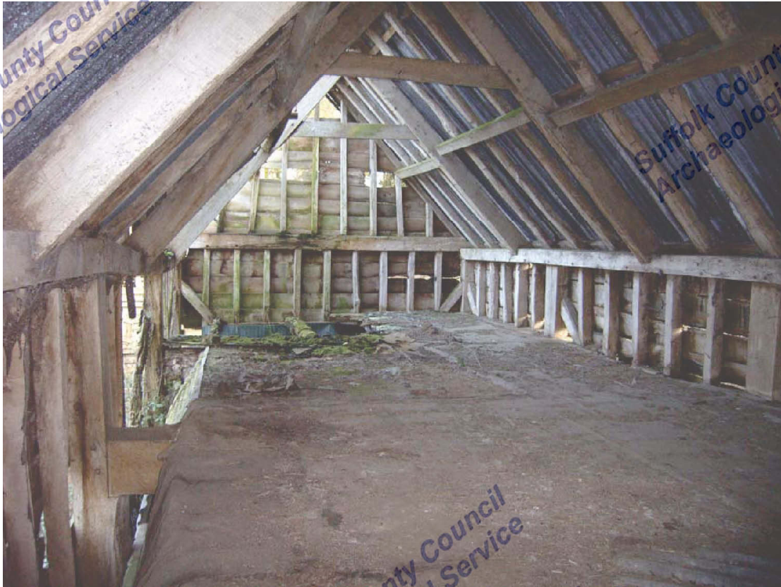
A2.11 Neathouse. Loft from west showing butt-purlin roof structure and loading vent above former hay rack against northern elevation to left
