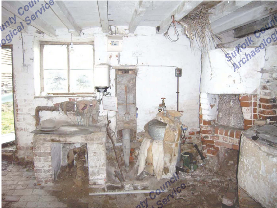
A2.9 Bakehouse. Interior of southern elevation showing stone sink to left, boarded pump in centre and oven to right
