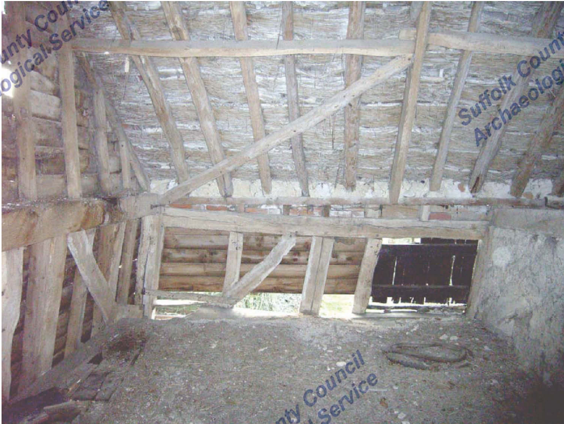
A2.17 Barn. Western internal elevation of stable loft showing original framed loading aperture to right
