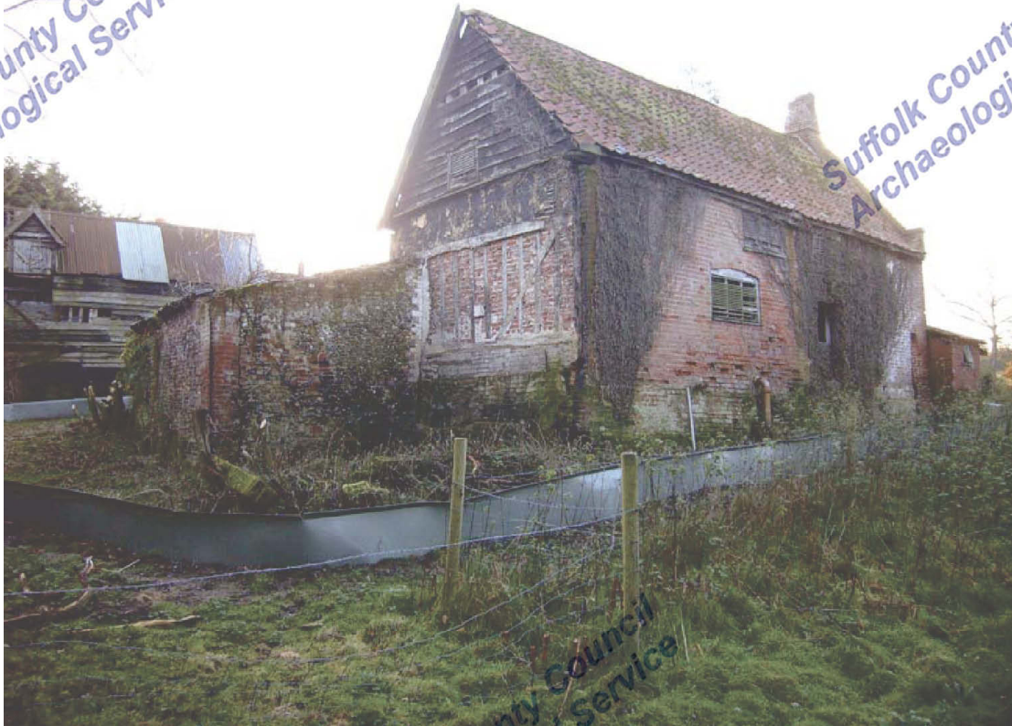
A2.5 Bakehouse. Exterior from north-east showing timber-framed eastern gable to left
