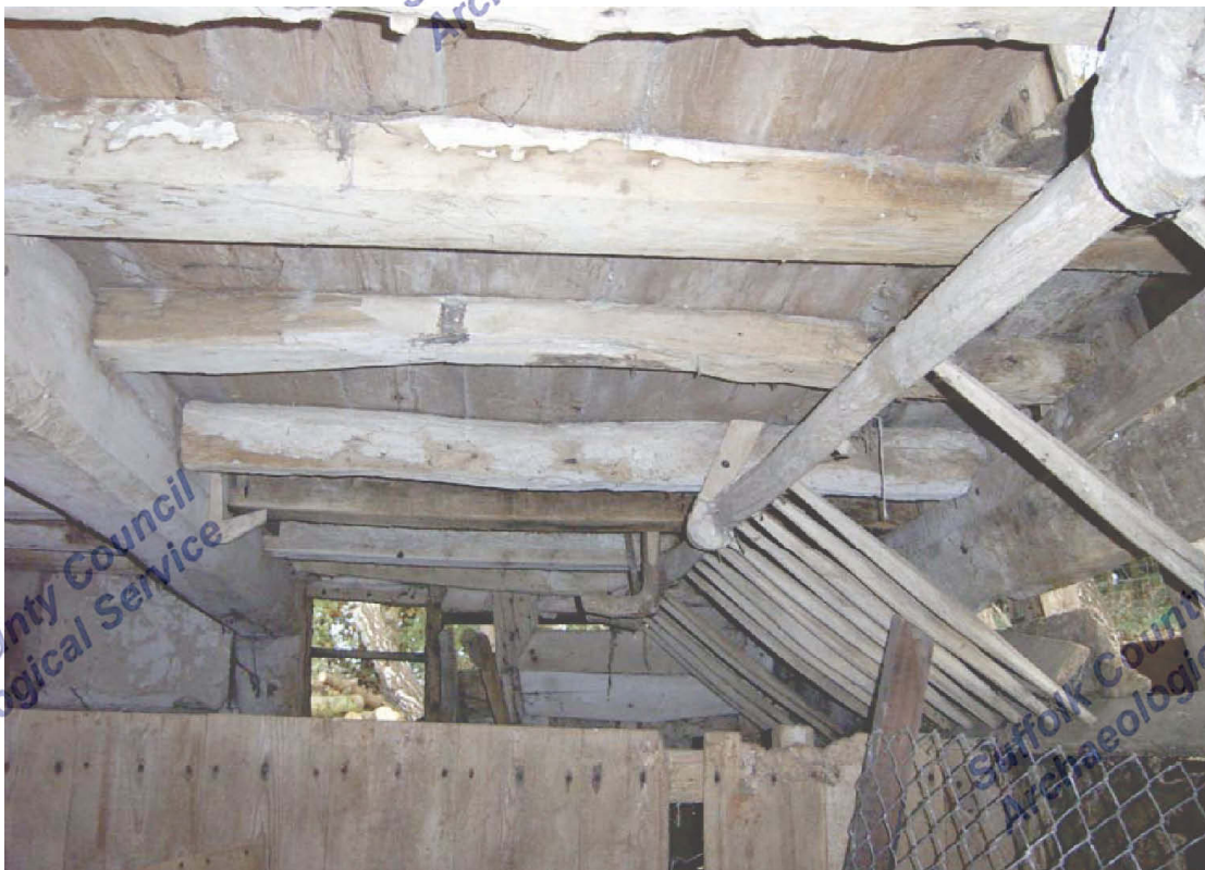
A2.16 Barn. Detail of stable ceiling from west showing hay rack against southern gable
