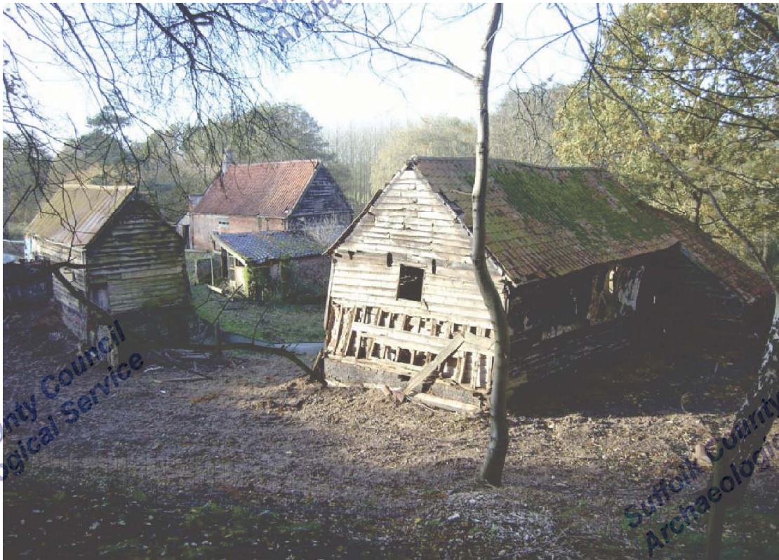
A2.2 General view of site from south-east showing barn to right (with attached stable in foreground), bakehouse in centre and neathouse to left
