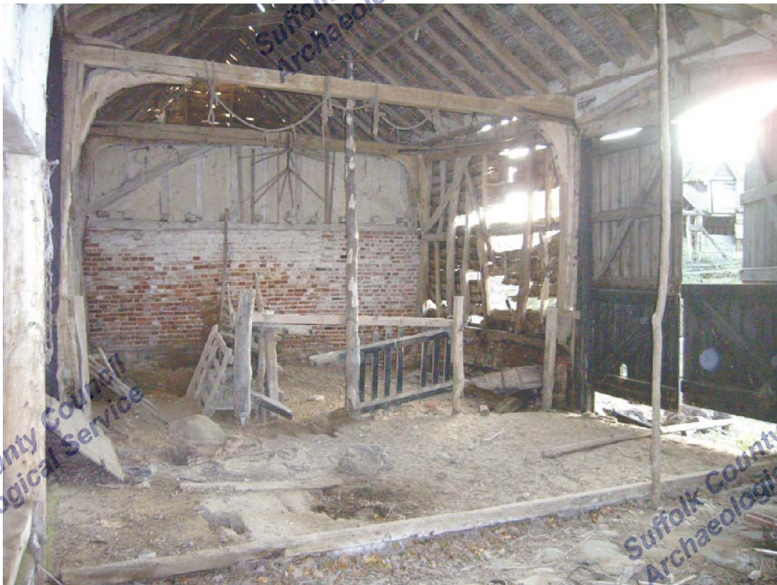
A2.14 Barn. General view of interior from north showing boarded threshing floor in central bay and secondary brick partition to stable in rear
