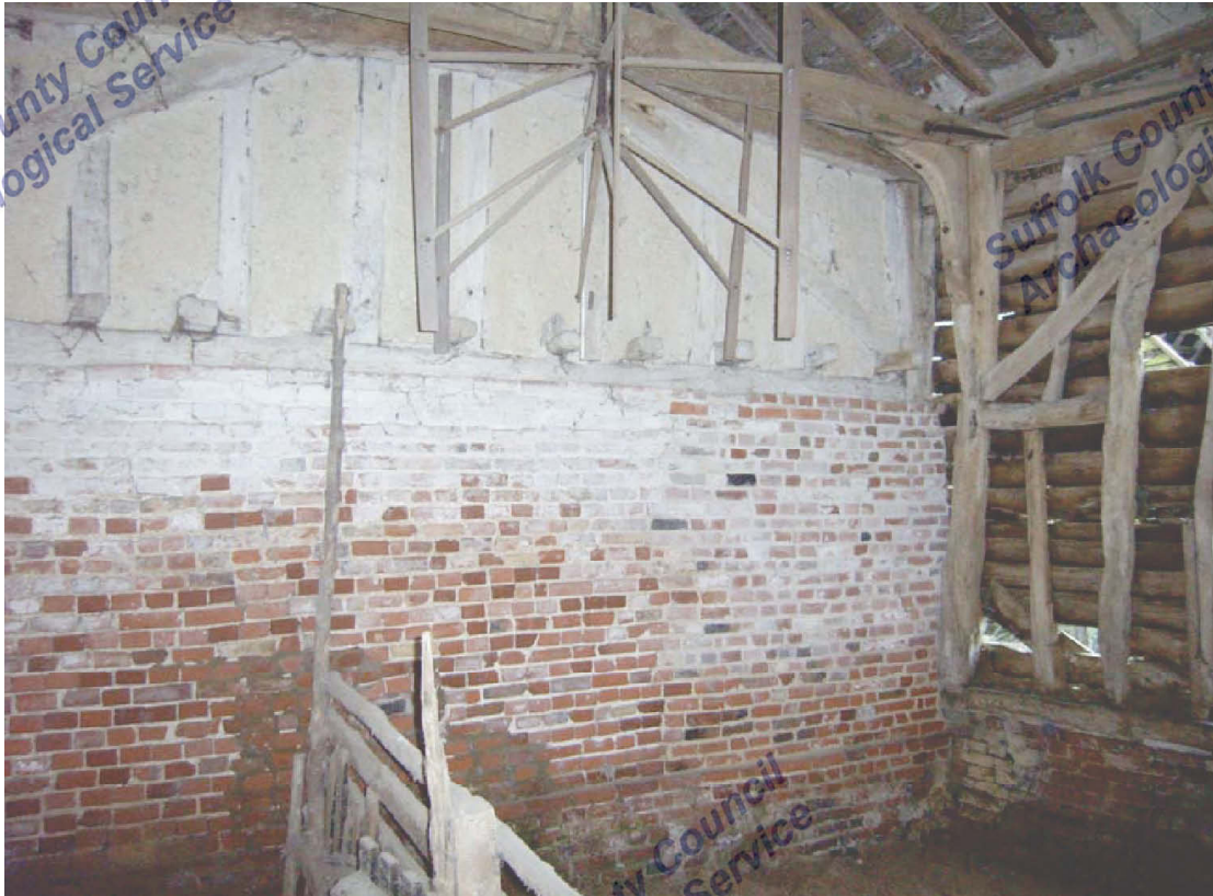
A2.15 Barn. Position of removed southern gable showing secondary brickwork to stable and original framing of three-bay barn with lintel of secondary door to right. The blades of a mechanical harvester hang from the tie-beam above
