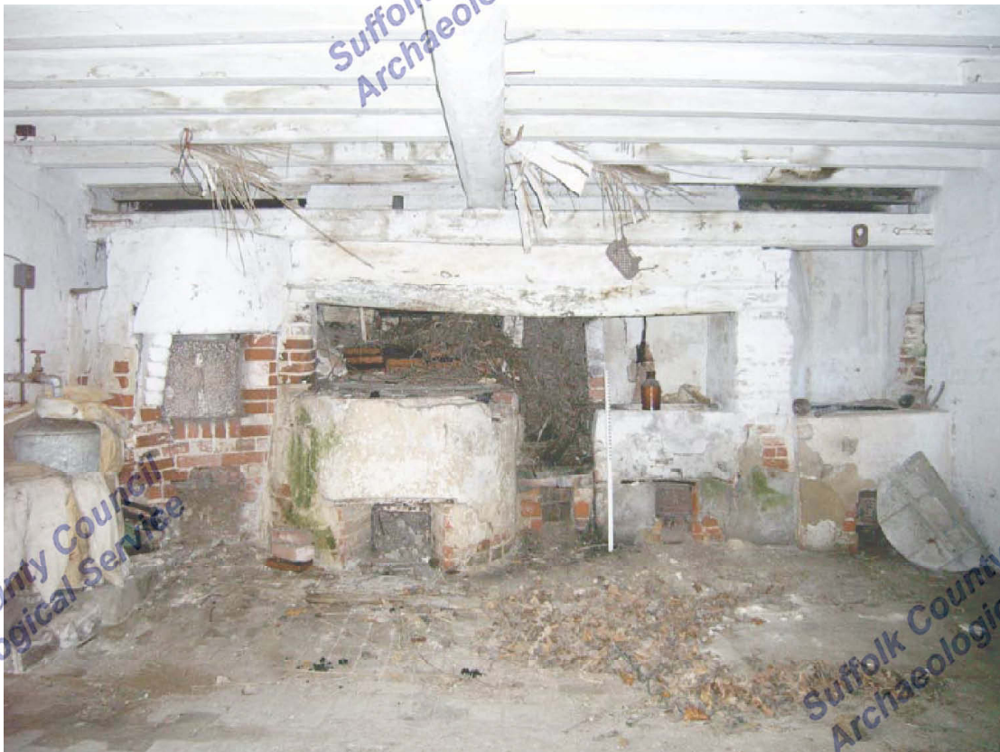
A2.6 Bakehouse. Interior of western gable showing chimney beam & three coppers to right with oven to left
