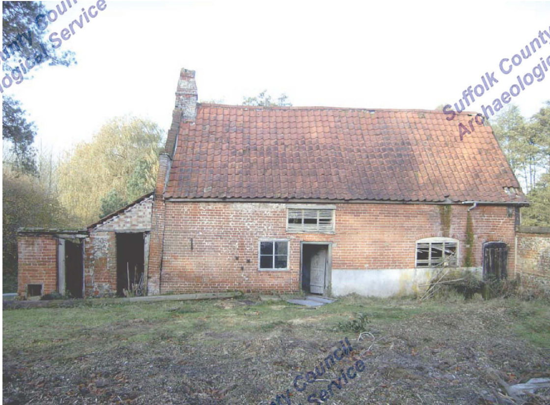
A2.3 Bakehouse. Southern external elevation with secondary brick façade showing central cross-entry with brick gable and integral chimney to left
