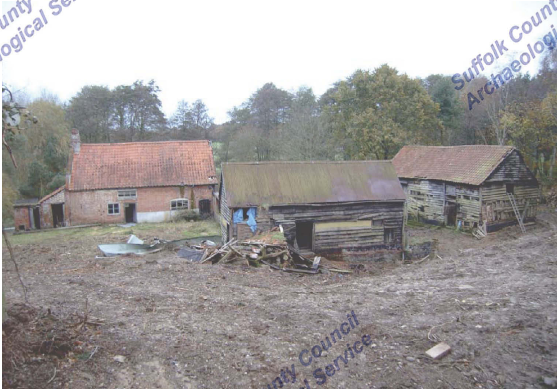
A2.1 General view of site from ridge to south showing bakehouse to left, neathouse in centre and barn to right
