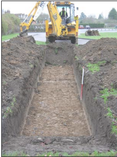
Plate 3 Trench 2 from the south-west
