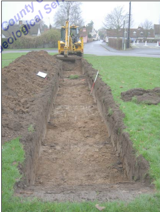
Plate 5 Trench 3 from the south-east
