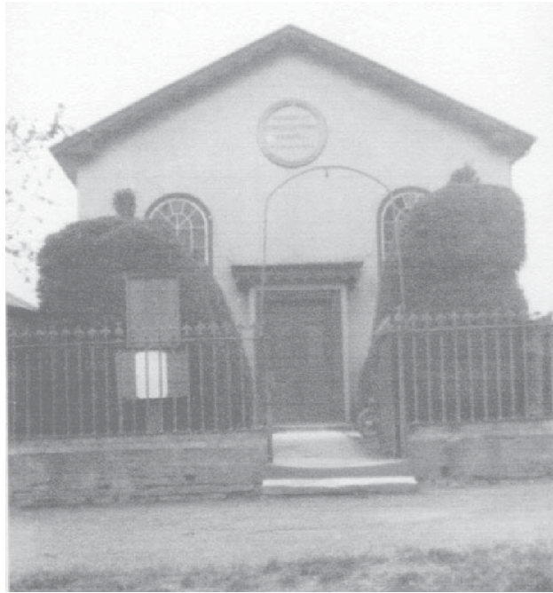
Figure 5 The northern gable in an old photograph (from a copy in the possession of the present owners)
