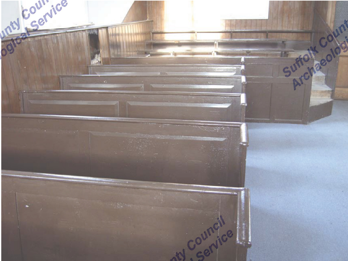
A2.9 Detail of chamfered boarded bench backs to western elevation (from south)
