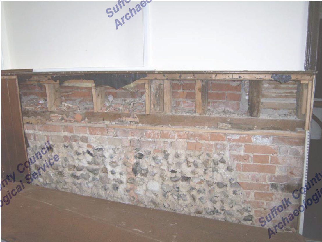
A2.10 Detail of flint plinth and studwork to interior of eastern elevation with vestry door to right
