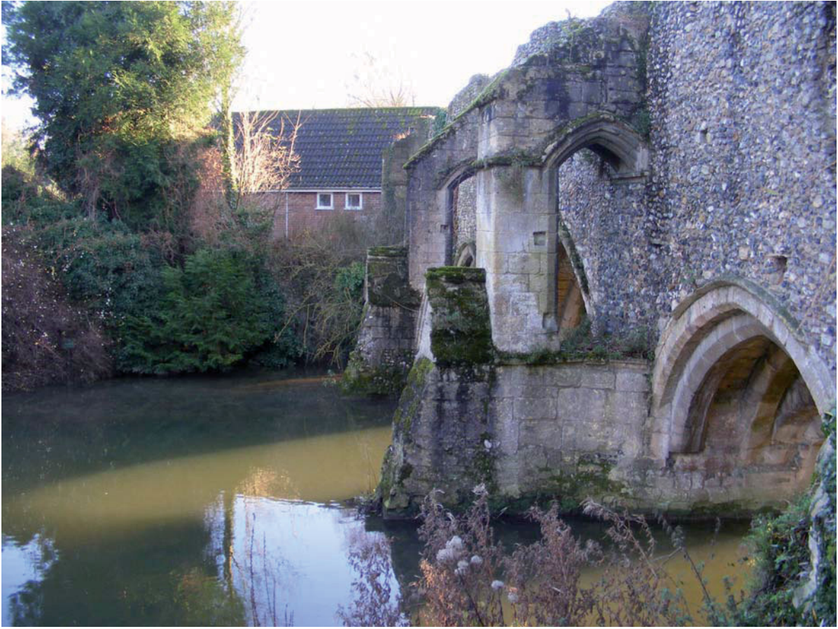
Figure 19. Abbot's Bridge and PDA viewed from the north
