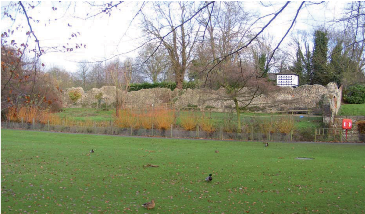
Figure 20. Abbey precinct wall viewed from the south west
