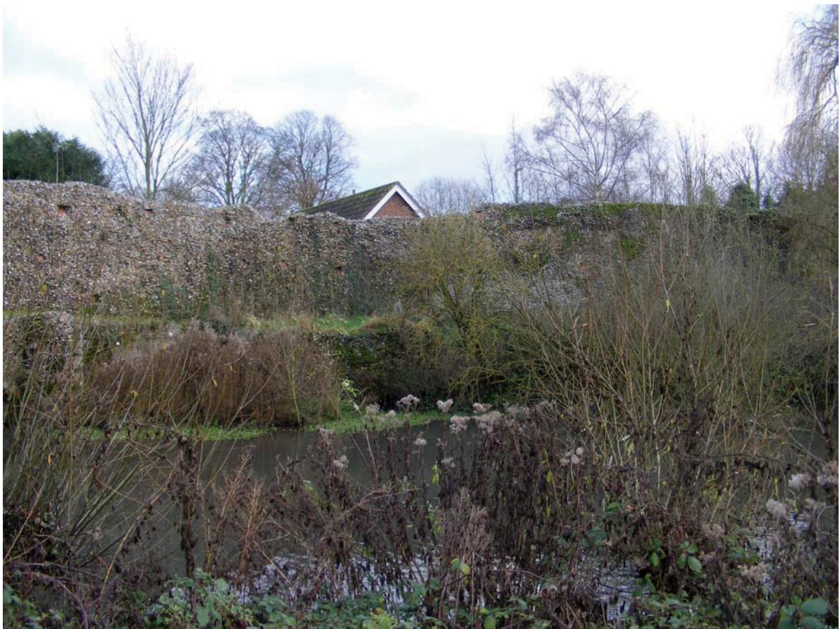
Figure 22. Abbey precinct wall viewed from the north west
