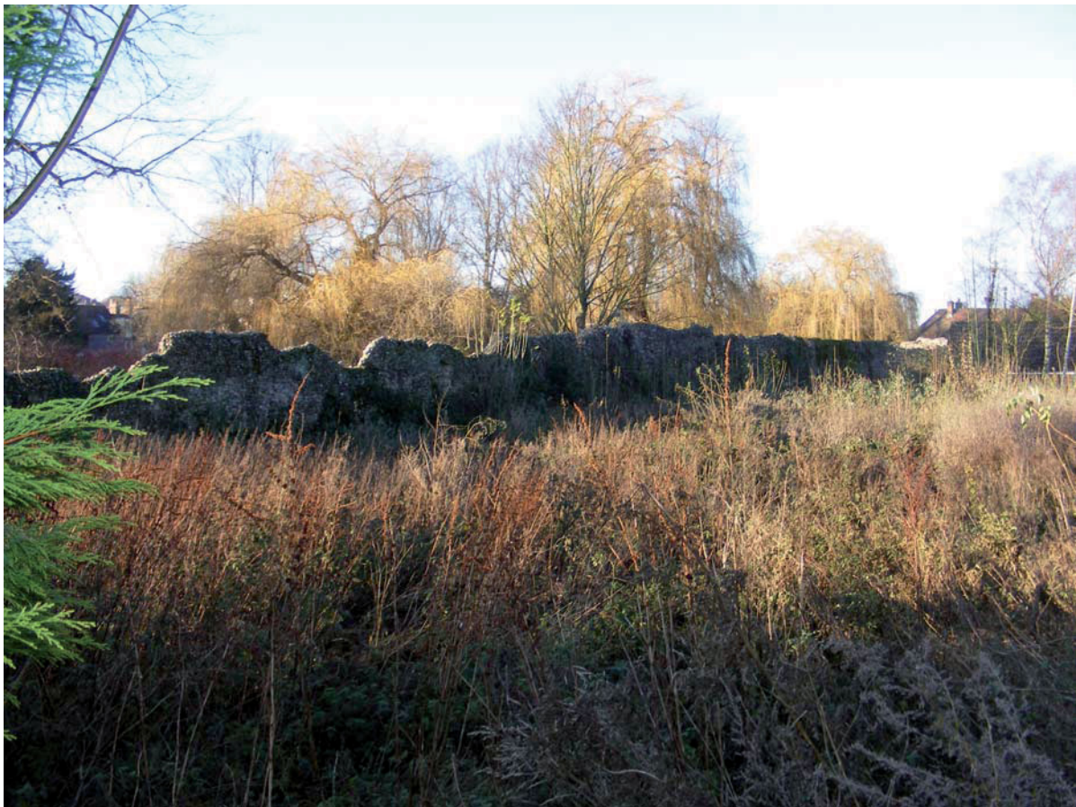
Figure 18. PDA and Abbey precinct wall viewed from the south east
