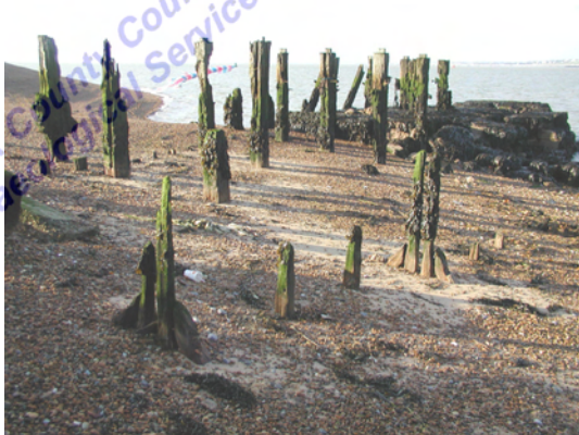
Pier and other timber structure remains
