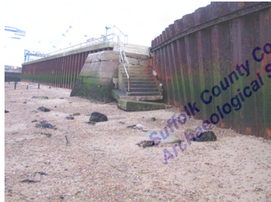
Pier stub (view looking north)
