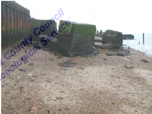
Concrete ?dolphin (view looking south)
