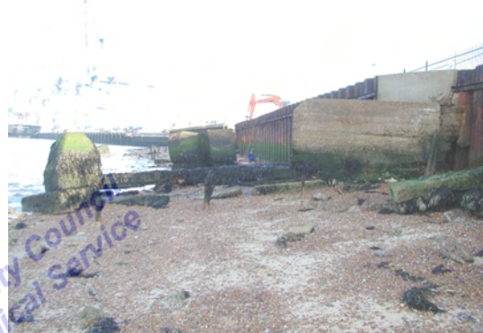
Concrete ?dolphin (view looking north)
