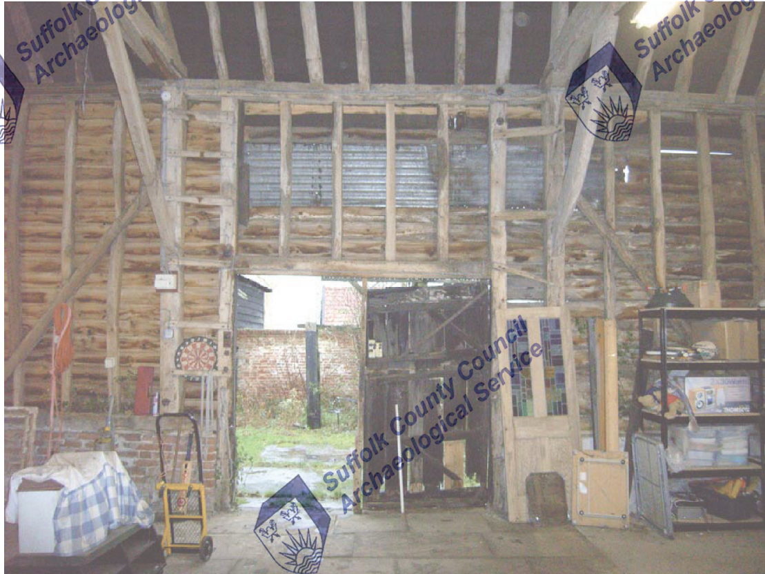
A2.5 Barn (1). Interior of central bay showing original wide, low door to west
