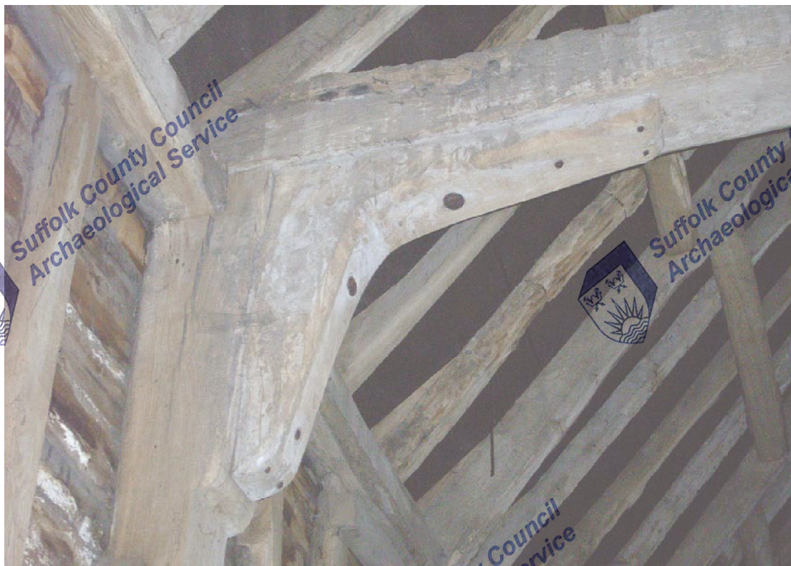
A2.4 Barn (1). Detail of the original jowl and bolted knee-brace in the open truss dividing the two northern bays, seen from the north
