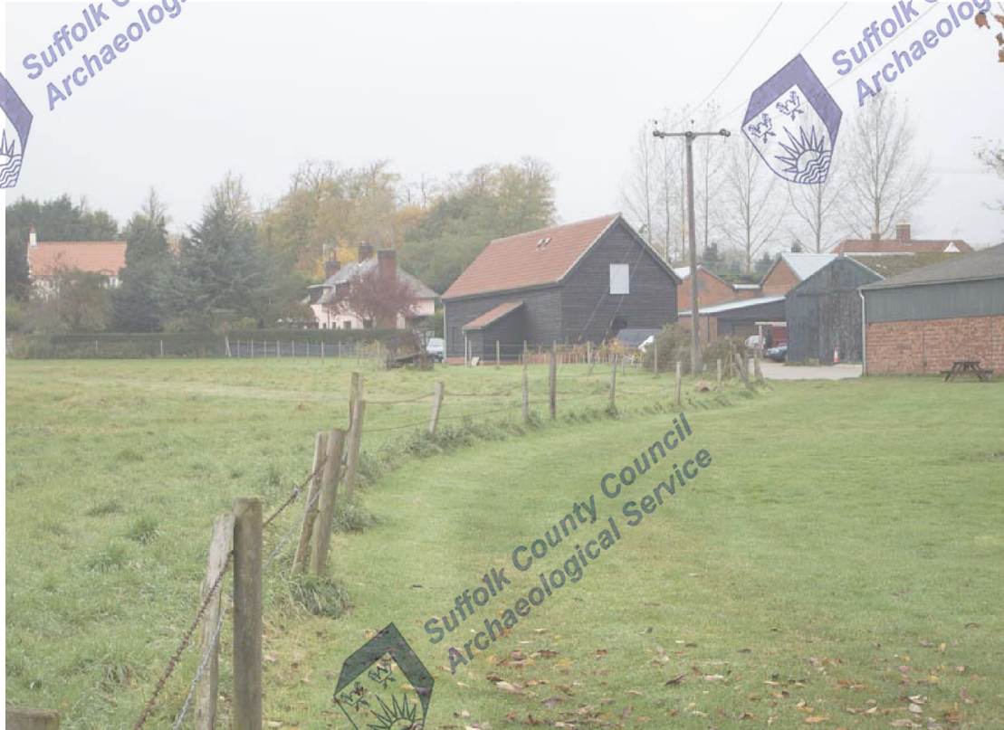
A2.3 General view from east showing from left to right Decoy Cottage, Decoy Farmhouse, recently erected weatherboarded 'barn', 19 th century yard buildings, roof of Decoy House (the original farmhouse) and 20 th century farm sheds
