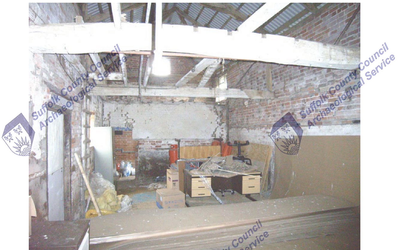
A2.8 Interior of stable (1). General view from west, showing remaining joists of removed hay loft with entrance to left and evidence of hay rack against southern wall to right
