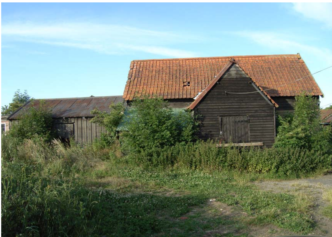
A2.2 Exterior of barn (1) from south-west showing shed (2) to left
