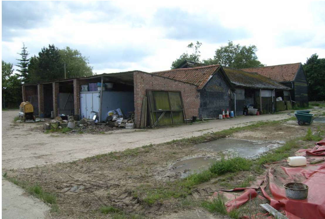
A2.3 General view of barn complex from north-east showing barn (1) to right and 20 th century brick shelter (6) to left.
