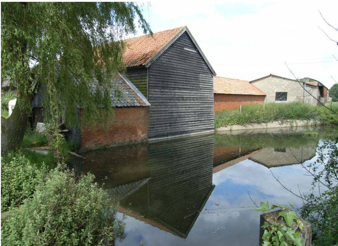
A2.2 General view of barn complex across pond from south-west, showing from left to right shed (2), barn (1), stable (3), block-work shed (9) and shelter shed (5)
