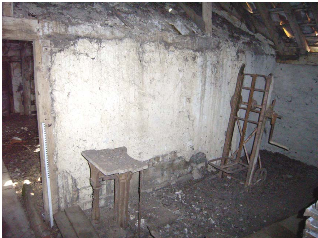
A2.14 Rendered external elevation of bays 6 & 7 from bay 13 showing first-floor door in bay 7 to left with weighing machine and sack trolley to right
