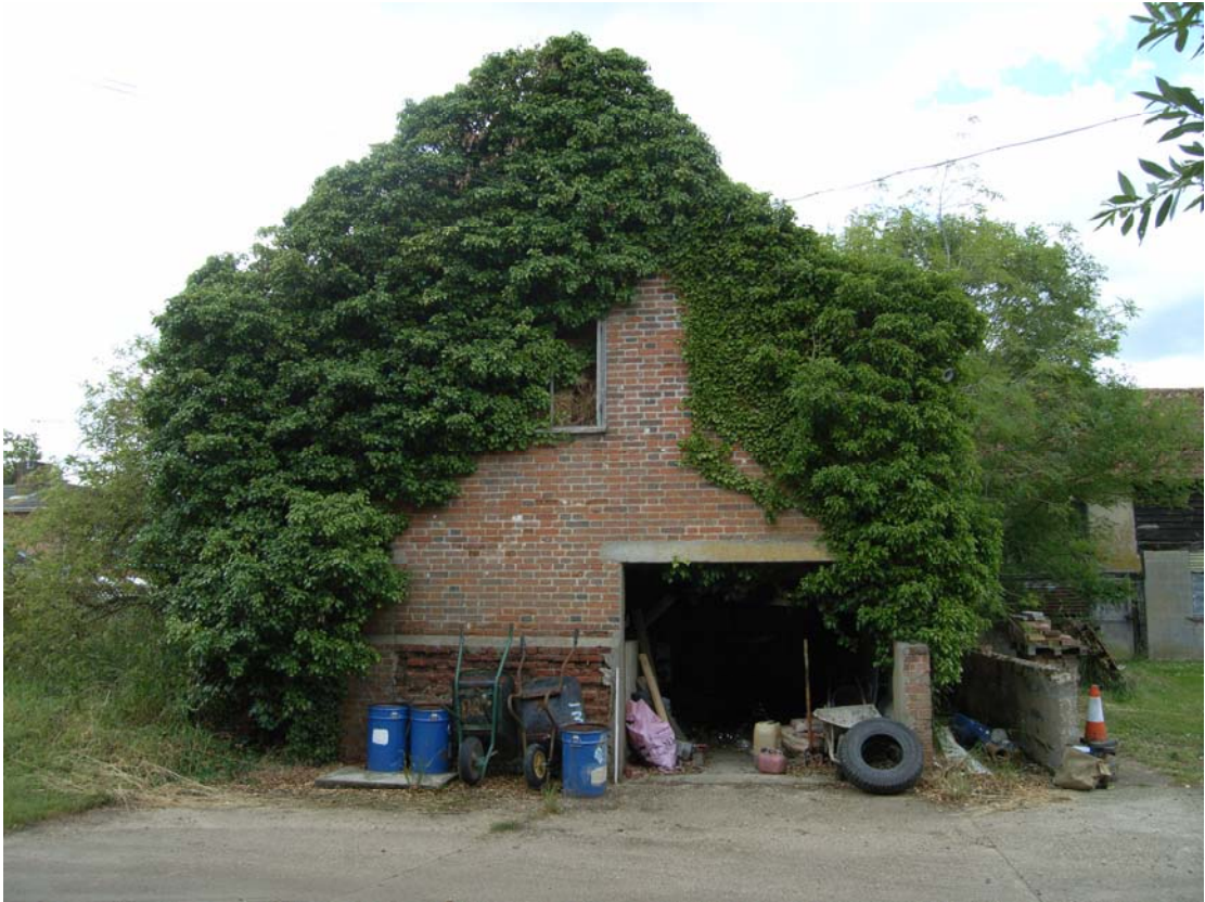
A2.3 Exterior of eastern gable showing secondary brickwork and entrance. Earlier brickwork at base shows signs of heat abrasion.
