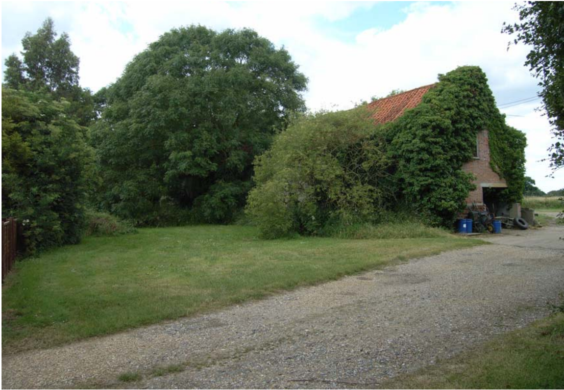
A2.1 General view of maltings from site entrance to south-east showing overgrown condition of main southern façade (rebuilt eastern gable visible to right)
