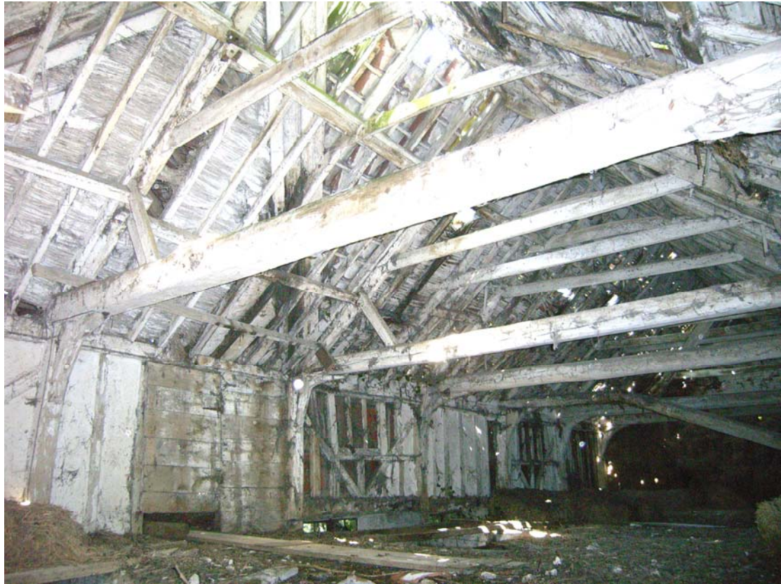
A2.13 Northern internal elevation of first floor showing bays 6-12 (left to right)
