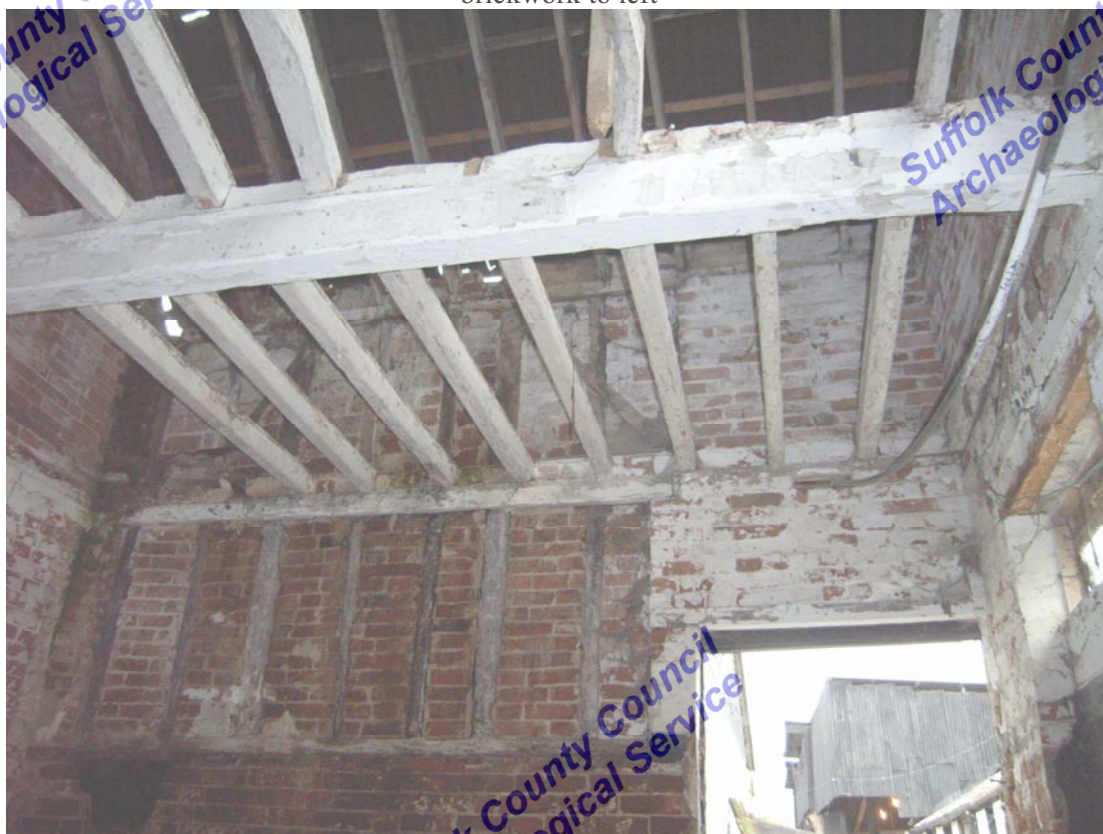
A2.7 Interior of northern shed (8) from east showing original external gable to left and joists of former loft. The western door is secondary.
