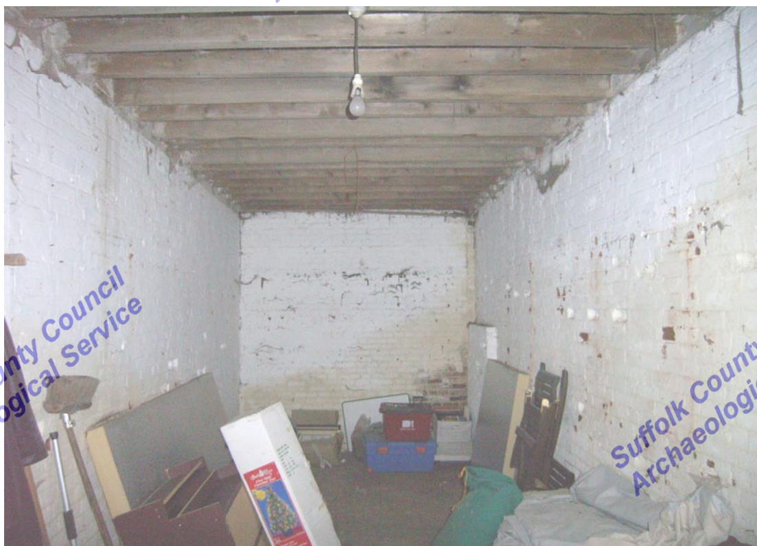
A2.7 Interior of northern shed (8) from east showing original external gable to left and joists of former loft. The western door is secondary.
