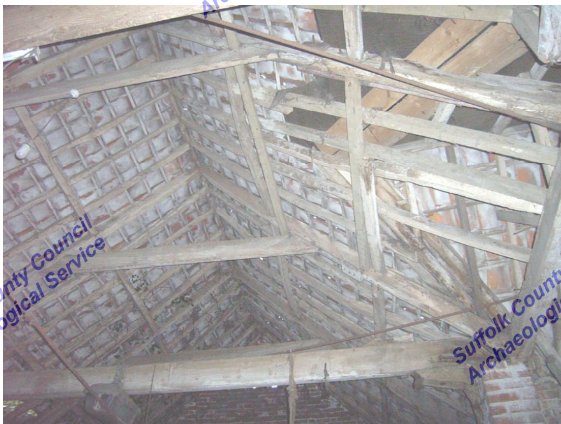
A2.9 Interior of shed (3) from south showing the original loft door in the northern gable above the renewed ceiling joists.
