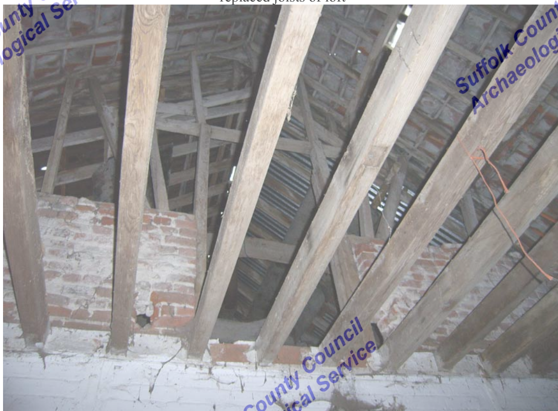
A2.9 Interior of shed (3) from south showing the original loft door in the northern gable above the renewed ceiling joists.
