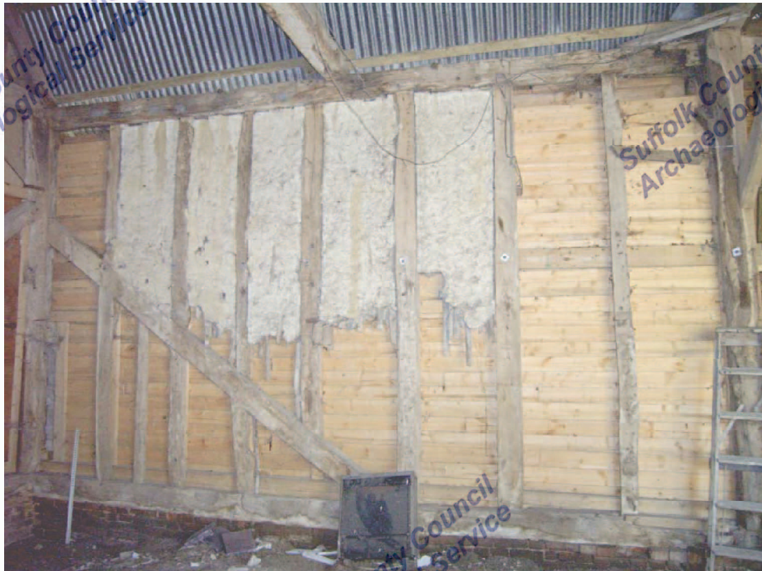
A2.5 Barn. Interior of rear (south-eastern) wall showing surviving panels of original wattle-and-daub infill with porch to right and north-eastern gable to left
