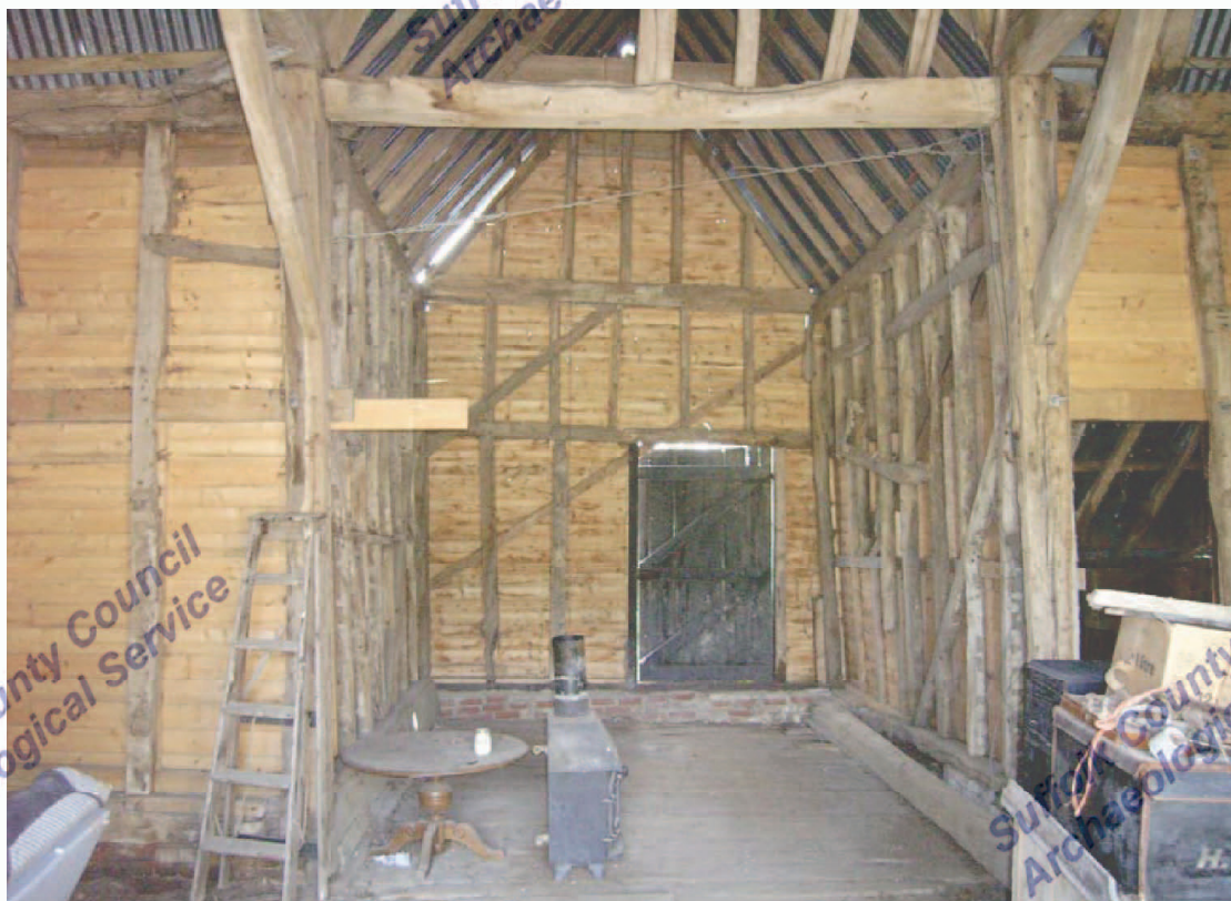
A2.6 Barn. Central bay with empty mortises of removed studs in roof-plate showing narrow later porch (2) with modern door in position of original wide door beneath original mid-rail
