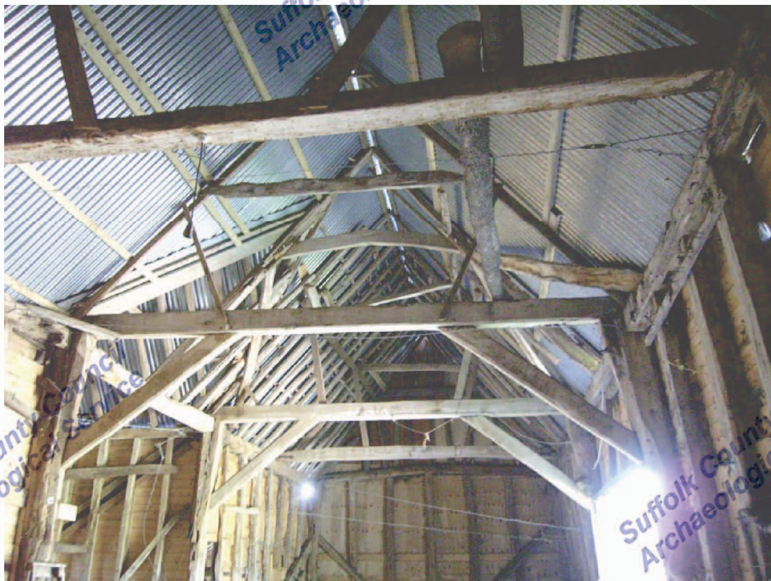
A2.4 Barn Interior. Roof structure from north-east showing original tie-beams, arch-braces and clasped-purlins
