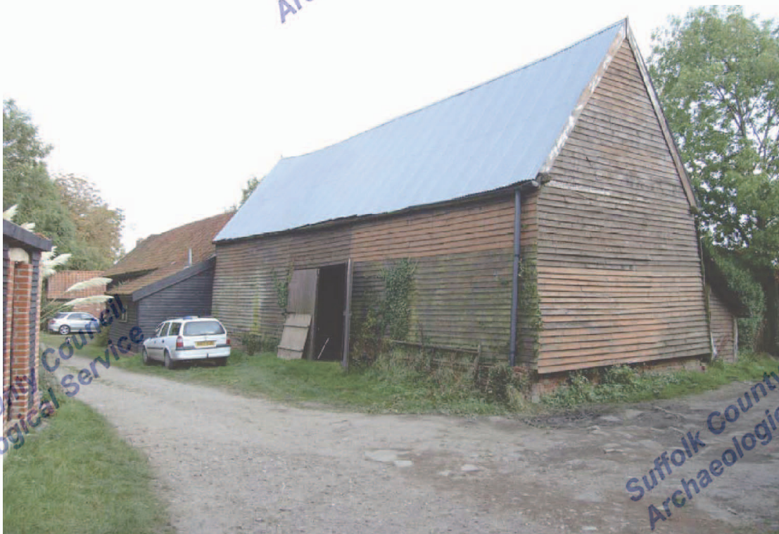
A2.2 Exterior of barn from west showing lean-to shed (3) to right and converted animal shed (7) to left
