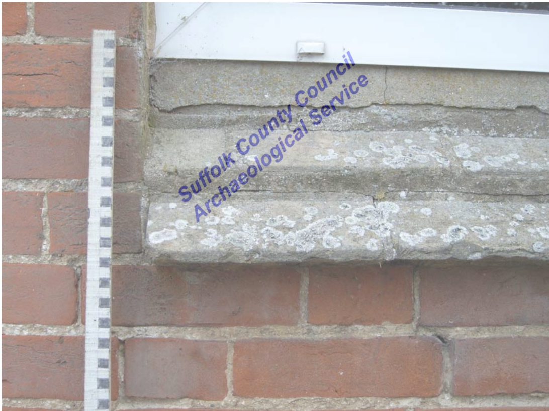
A2.4 Detail of original moulded gault brick window sill in eastern elevation
