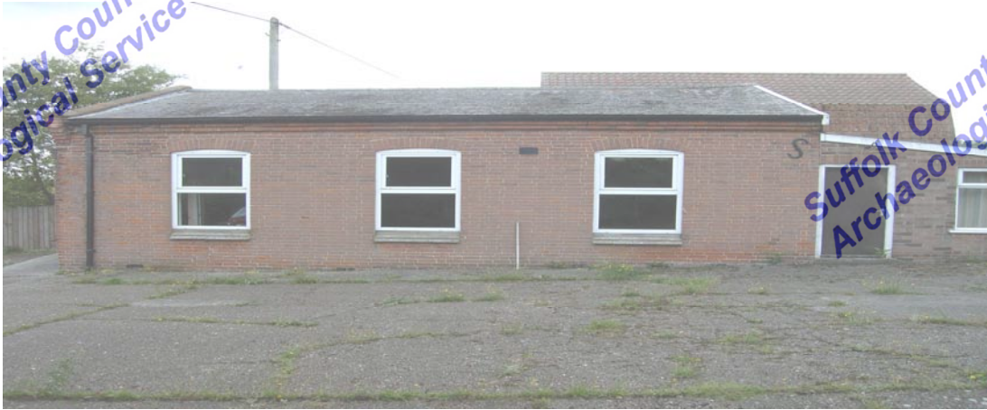
A2.3 Eastern external elevation showing recently replaced windows with 20 th century extension (3) to right.
