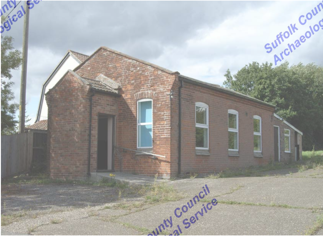
A2.1 Exterior from south-east showing pedimented arch of original entrance in southern gable just visible above 20 th century porch (4)
