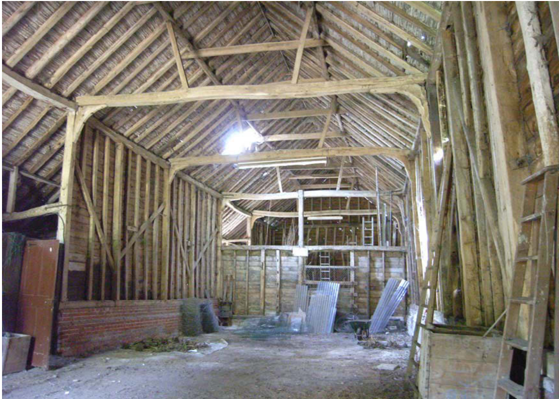
A2.9 Interior of barn. General view looking west from eastern gable. The original structure ended at the partition between bays C & B shown here in the rear and was later extended westwards by two bays.
