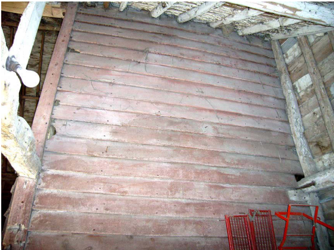
A2.8 Rare reddled external boarding to bay C of barn from later lean-to shed G
