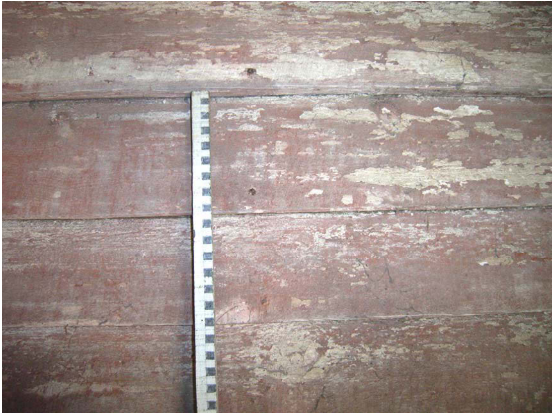
A2.7 Detail of original reddled external boarding to barn preserved within later shed H
