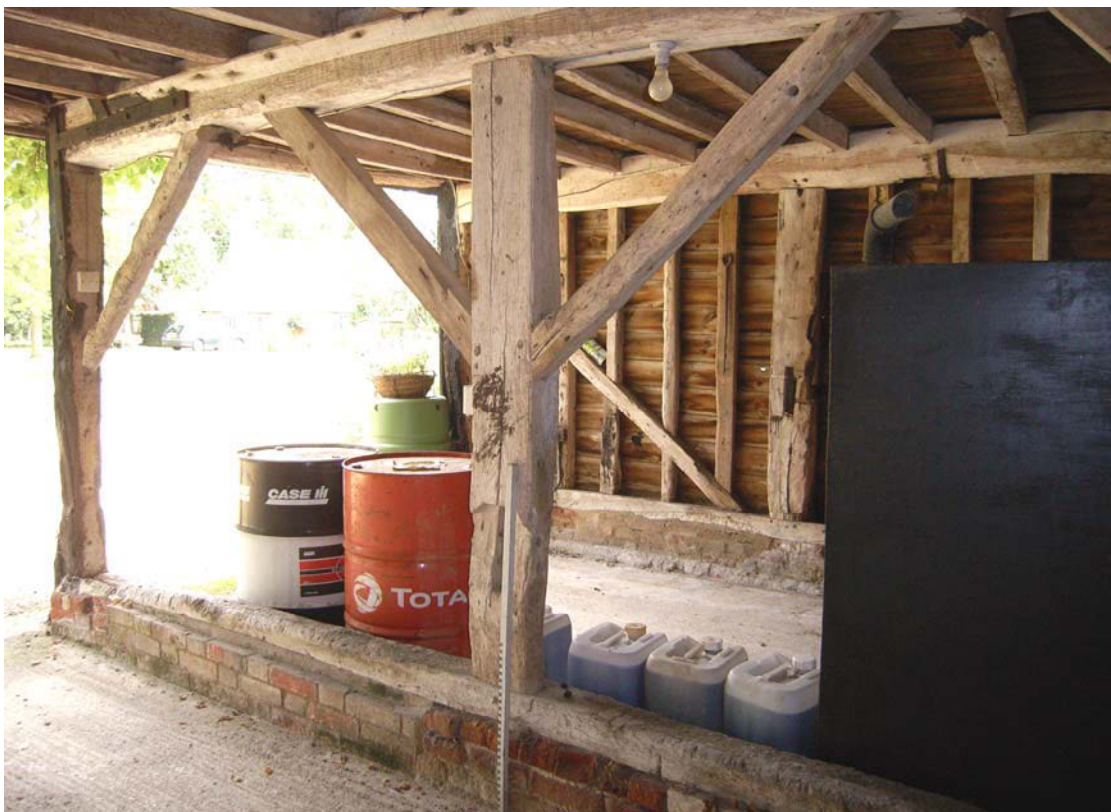
A2.10 Interior of cartlodge (2) from north-west showing open bays & re-used timber
