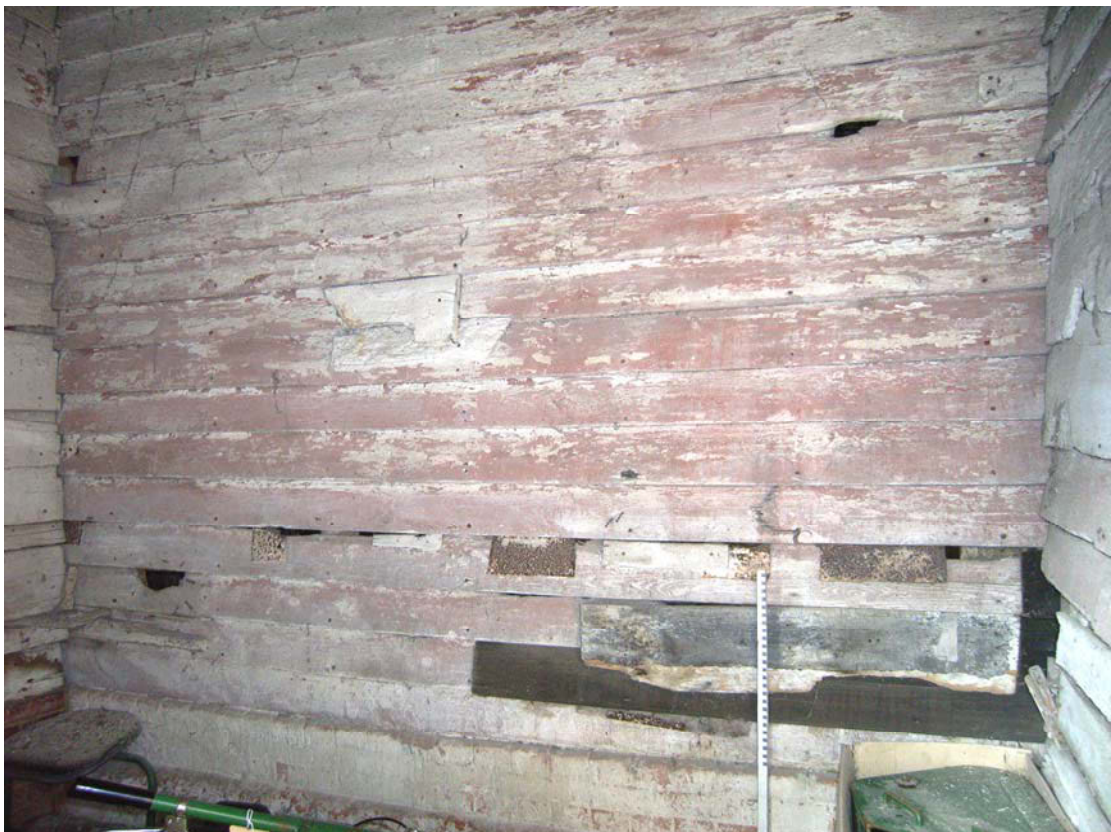
A2.6 Interior of shed H from south showing rare original reddled external boarding to barn beneath later whitewash
